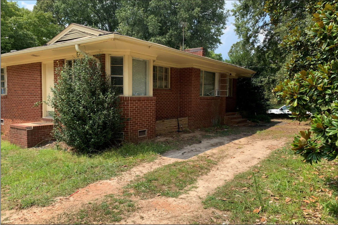
Photo 19: 1011 Oberlin Rd, Raleigh, NC (08/10/2021) Perspective view of the south side of structure from adjacent property on Oberlin Rd, facing northwest.
