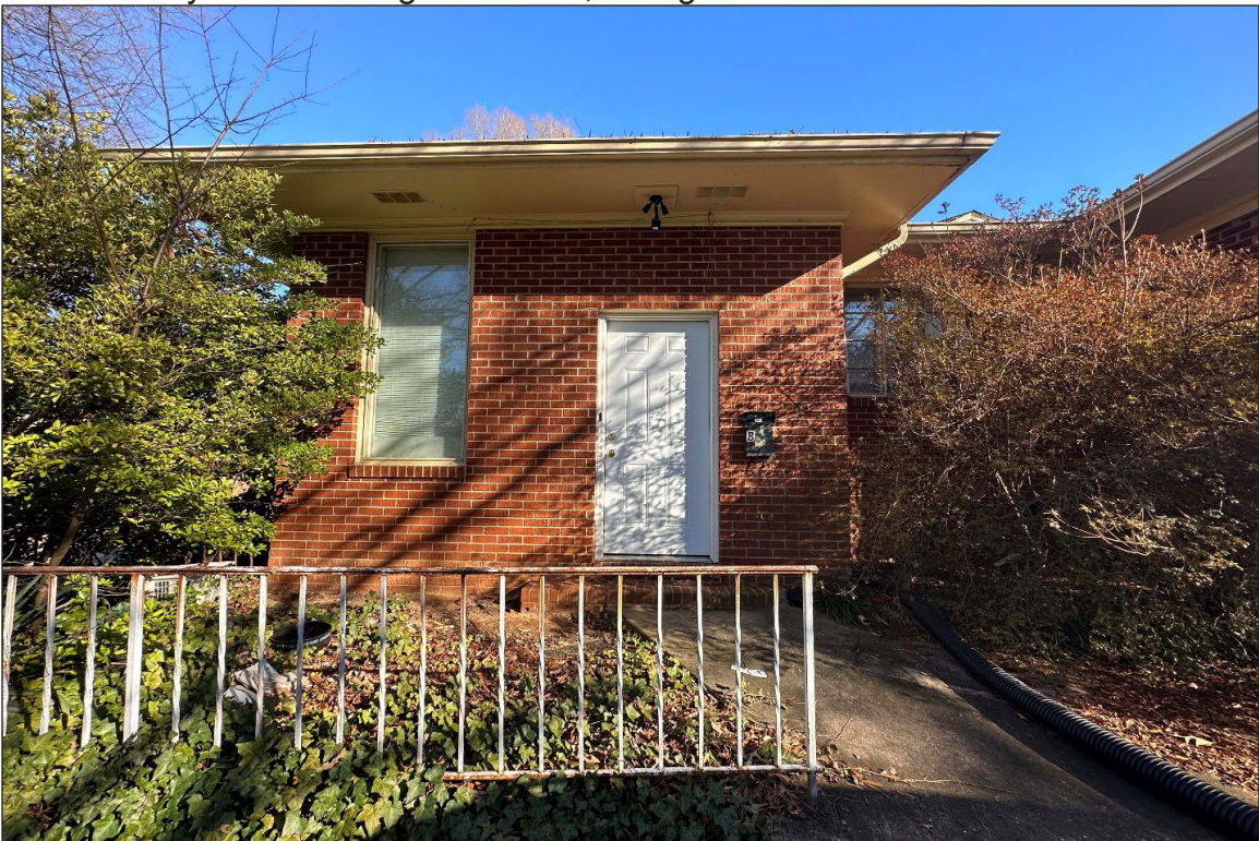
Photo 10: 1011 Oberlin Rd, Raleigh, NC (01/10/2023) Partial west elevation showing addition on left and original structure on right, facing east.
