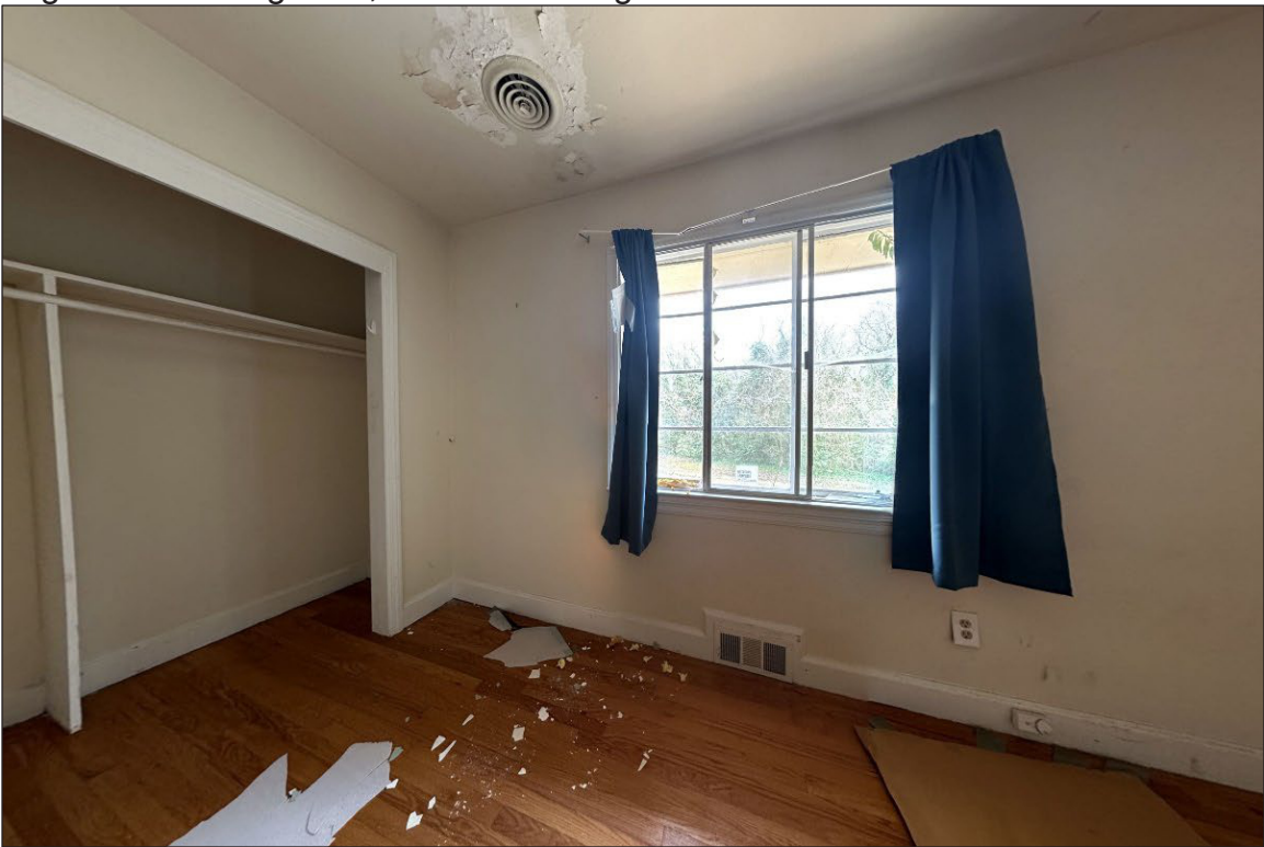
Photo 28: 1011 Oberlin Rd, Raleigh, NC (01/10/2023) Interior photo of hall bedroom facing south showing casing and steel casement window.
