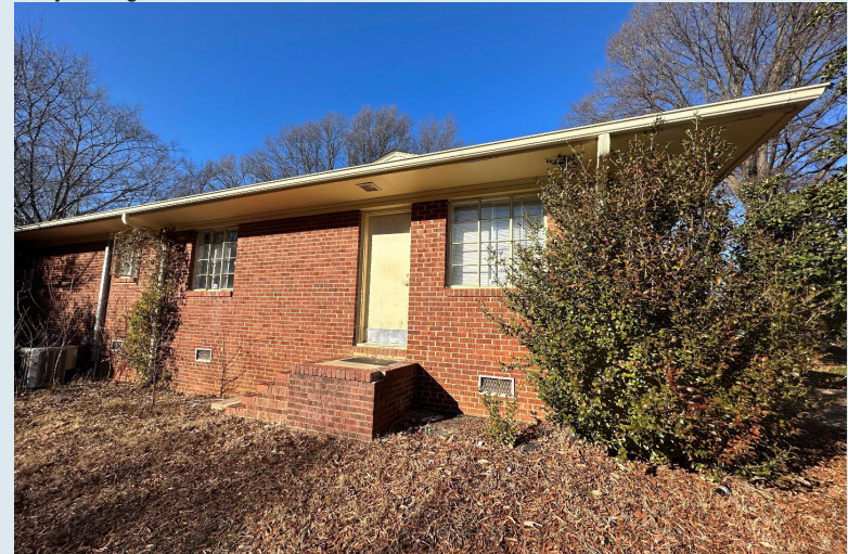
Photo 02: 1011 Oberlin Rd, Raleigh, NC (01/10/2023) Southeast corner showing larger overhang, facing north.
