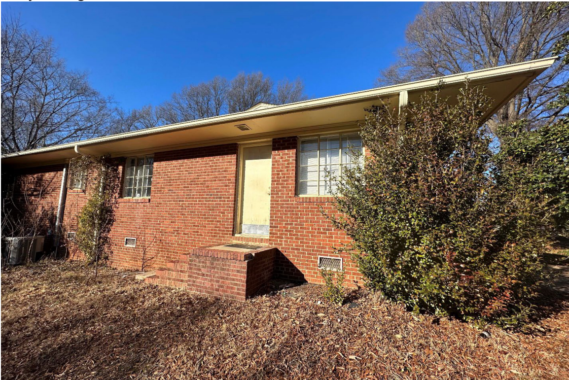
Photo 02: 1011 Oberlin Rd, Raleigh, NC (01/10/2023) Southeast corner showing larger overhang, facing north.
