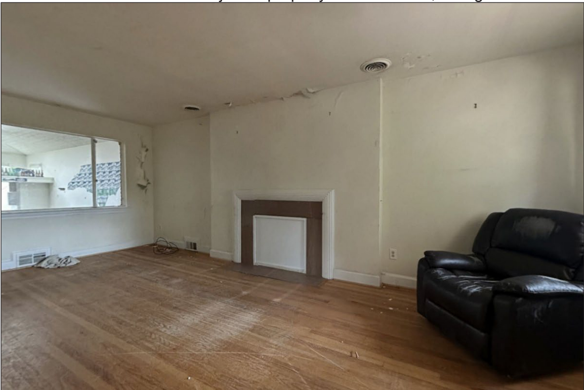
Photo 20: 1011 Oberlin Rd, Raleigh, NC (01/10/2023) Interior photo of front living room, facing north wall at original fireplace, brick has been drywalled/plastered.
