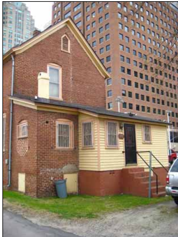
Rear shed detail
