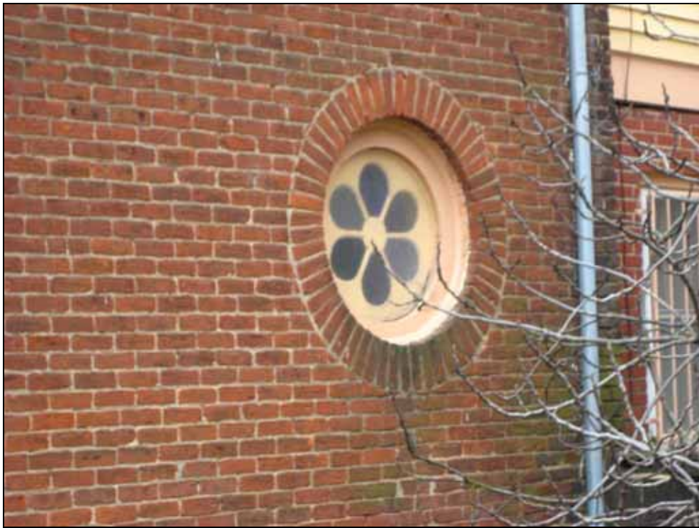
Circular window detail (north/side elevation)
