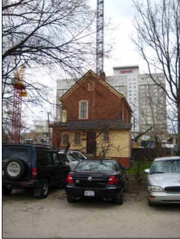
Site view from rear elevation (looking west)
