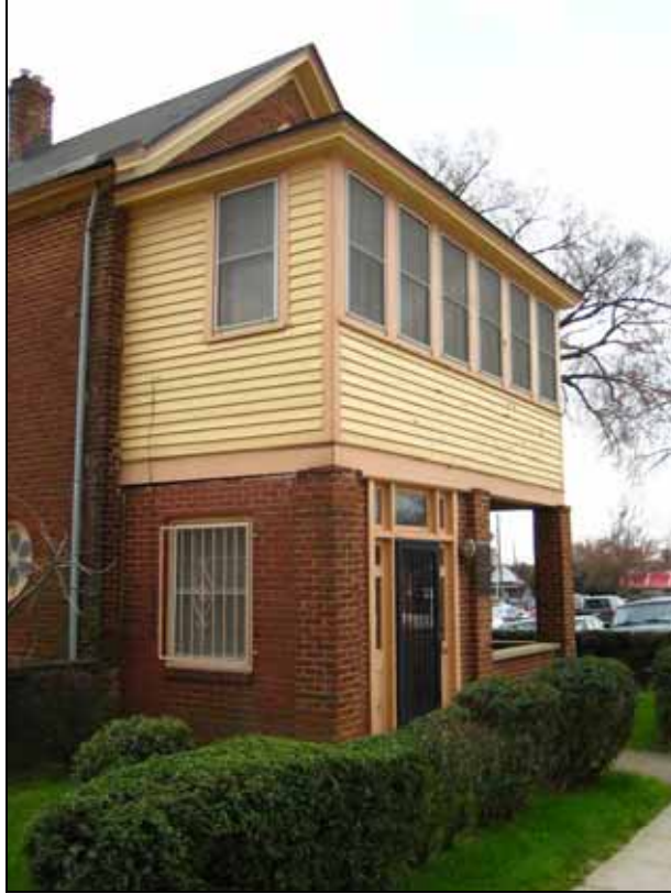
Façade view (looking at NW corner)
