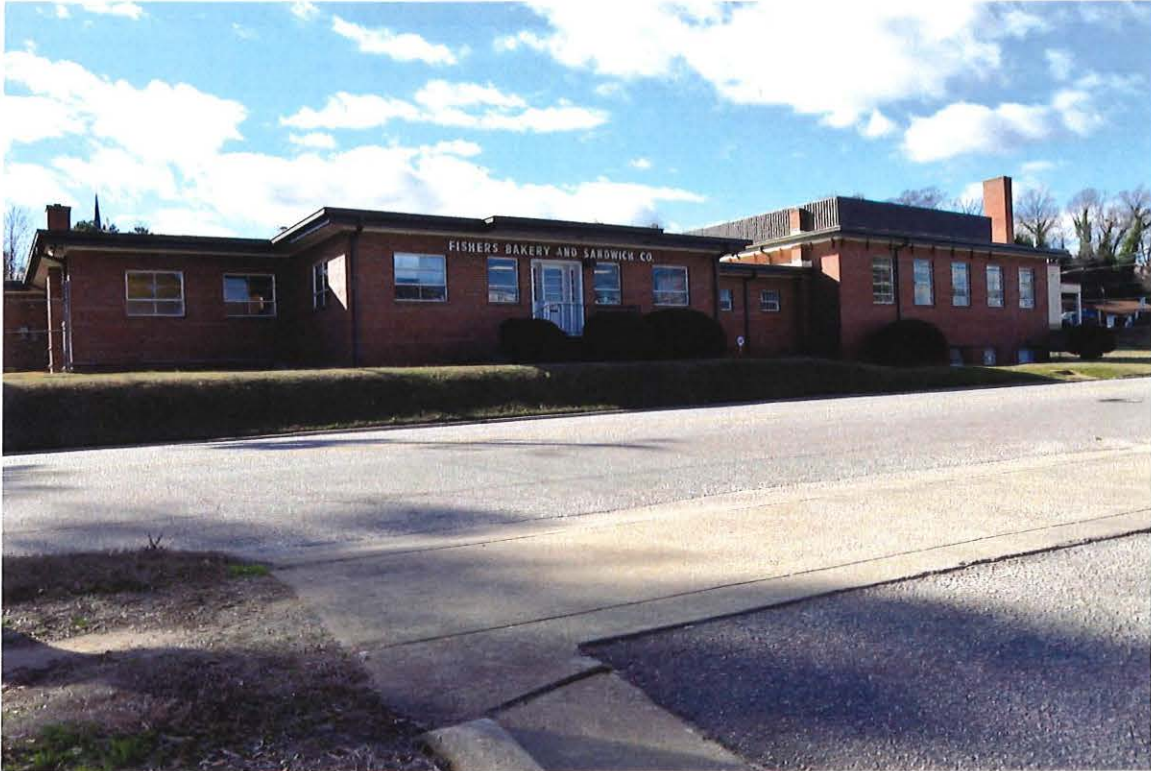
Fisher's Bakery & Sandwich Company, facade, view SW.
