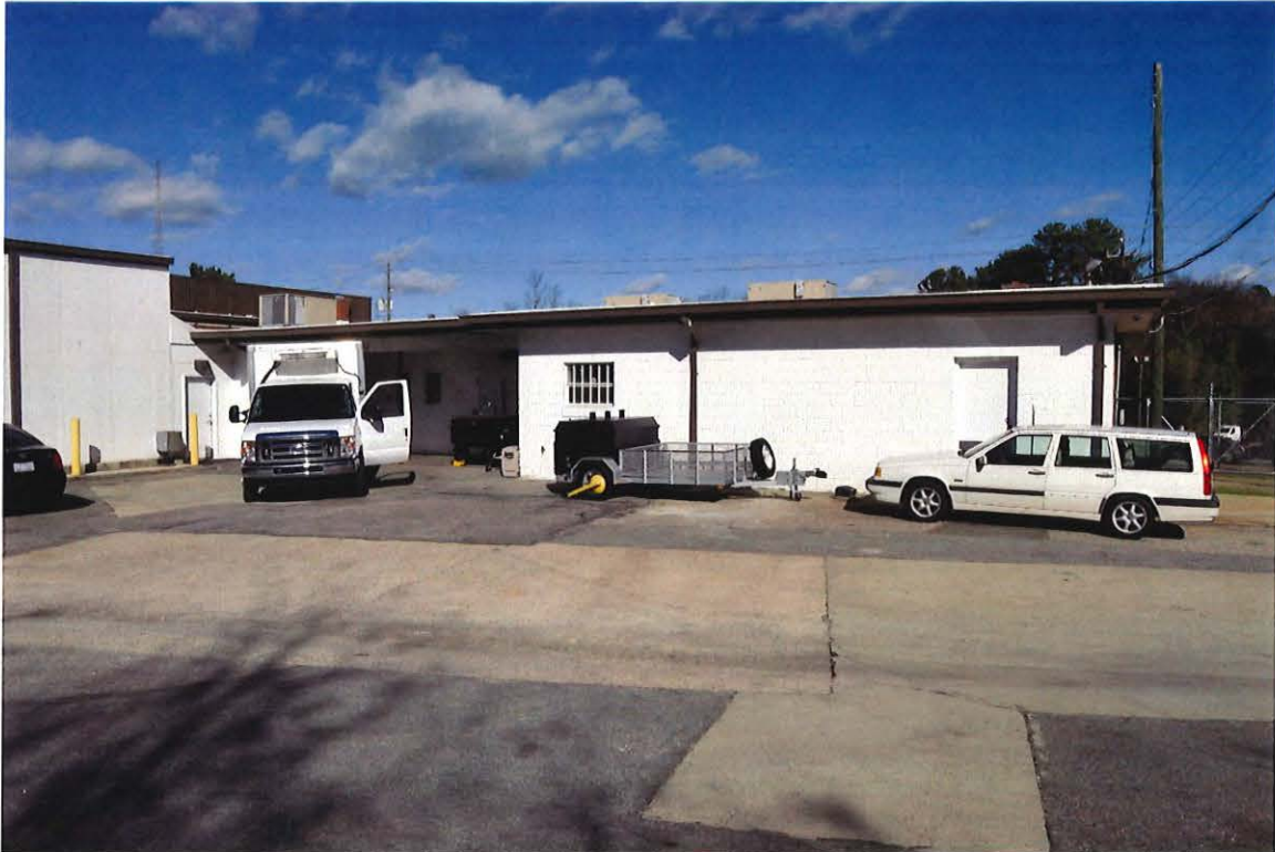
Fisher's Bakery & Sandwich Company, rear elevation, view N.
