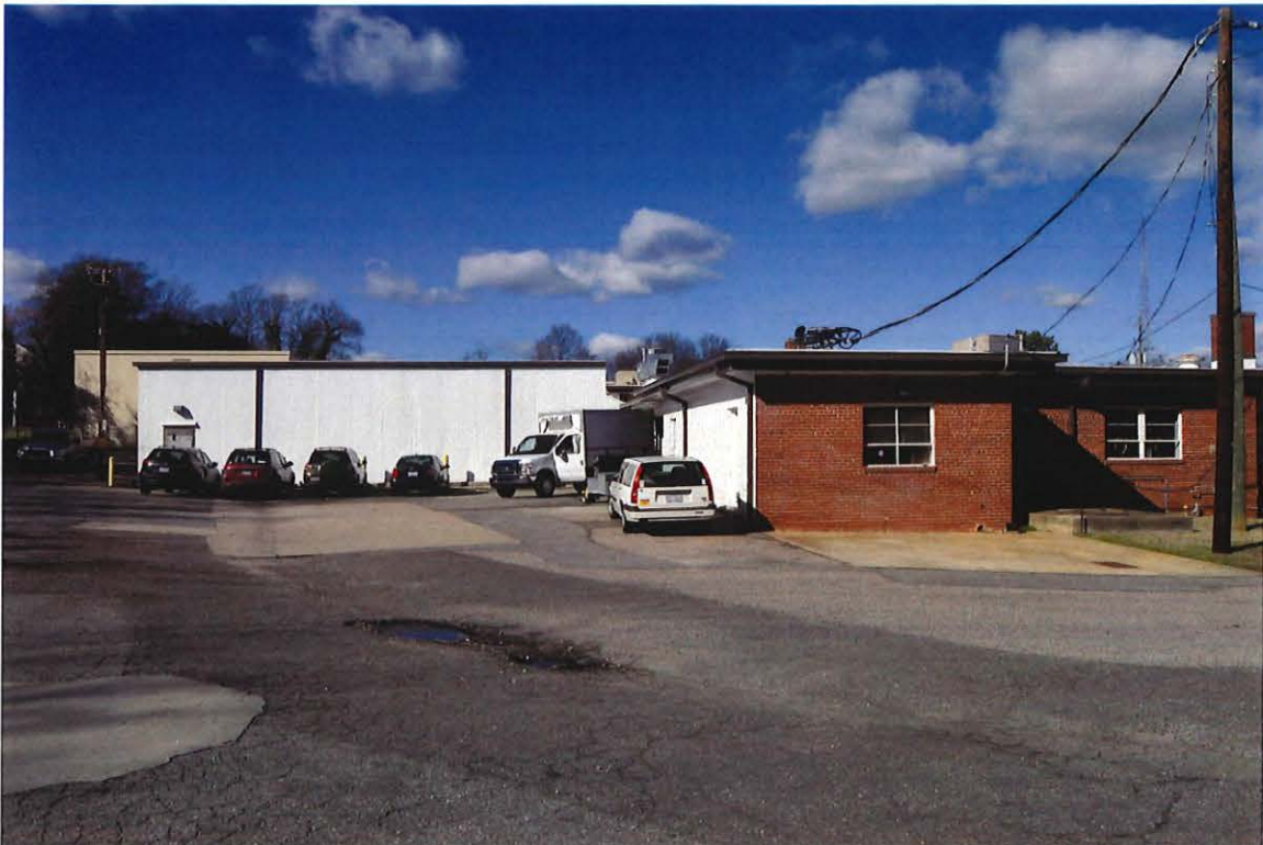
Fisher's Bakery & Sandwich Company, rear refrigeration rooms, view W.
