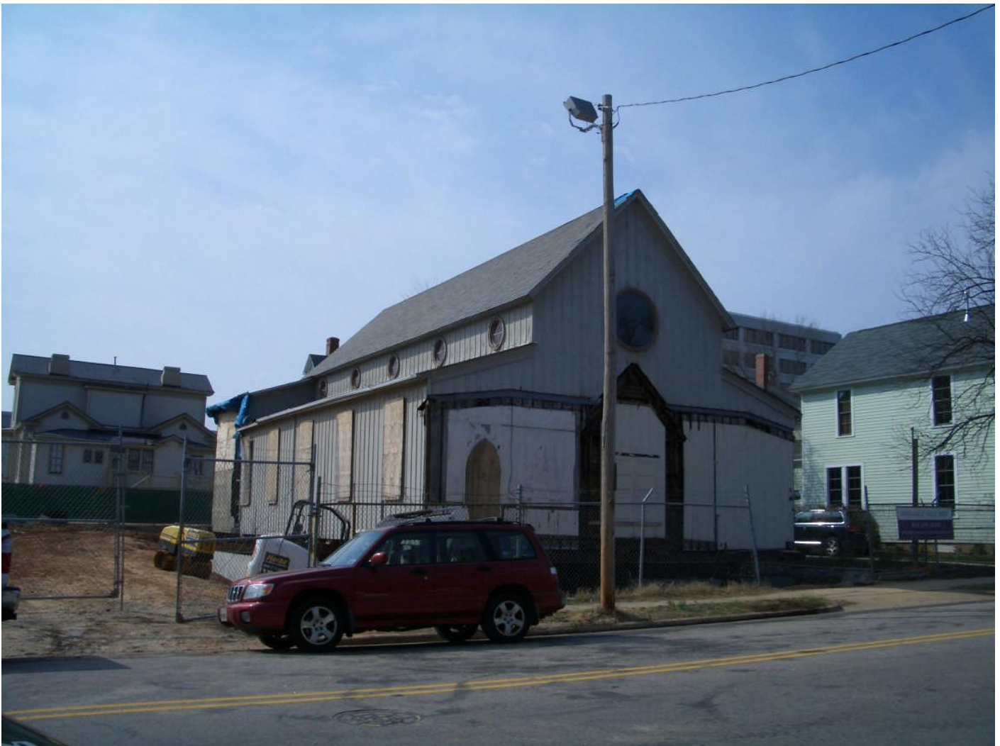
Fig. 6. All Saints Chapel exterior, 110 S. East St., Raleigh. March 2007. (photo by M. Ruth Little)
