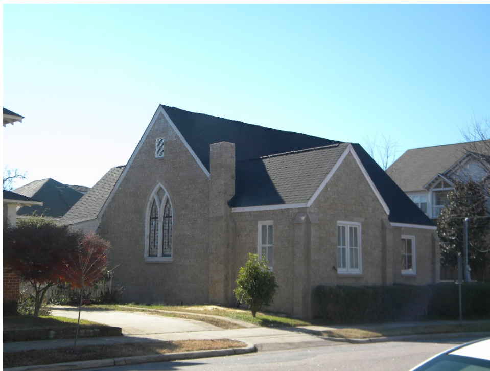
Figure 5. East elevation with north wing and the stained glassed gothic arch window shown.
