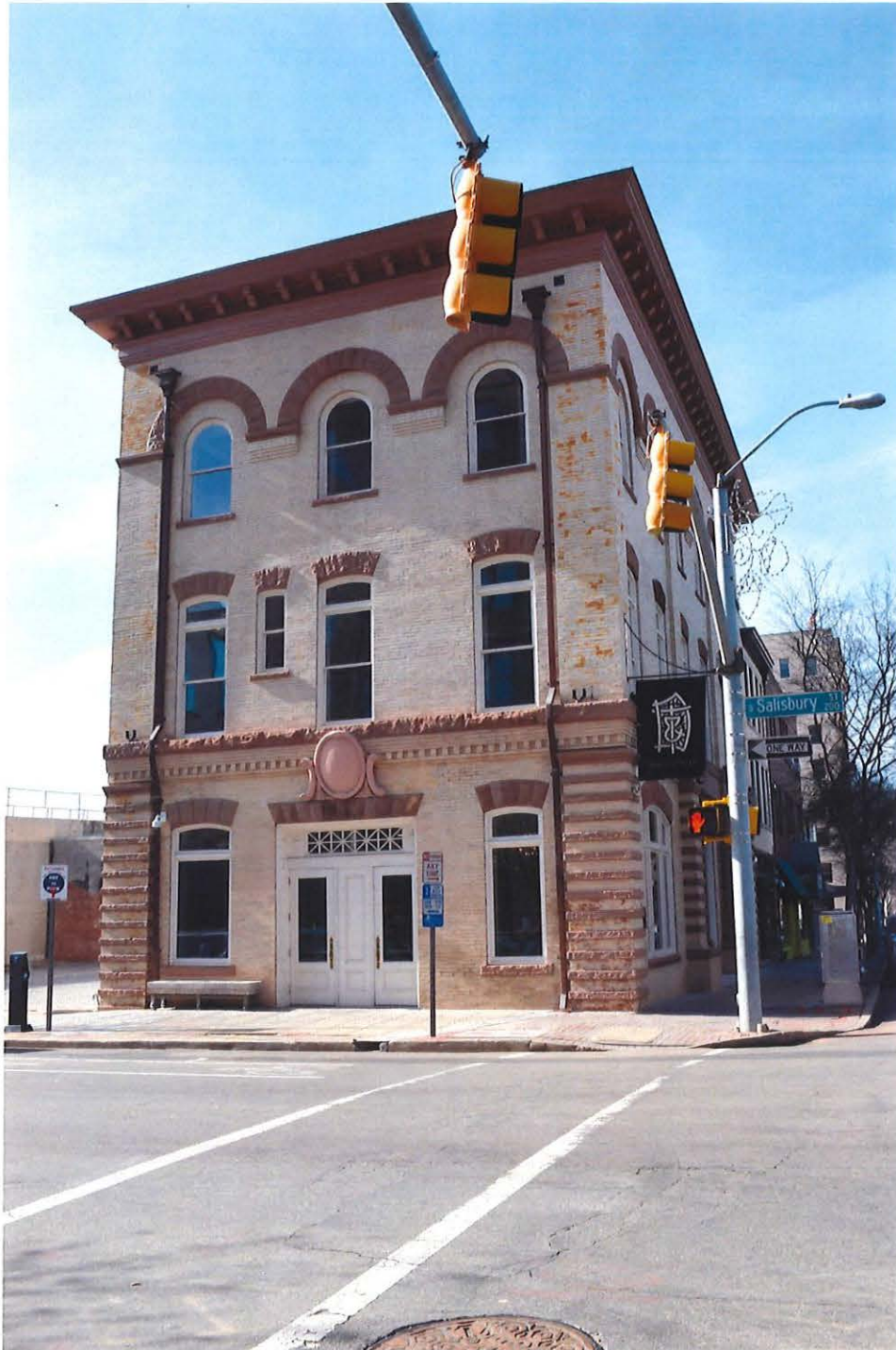
H. J. Brown Coffin Company, east elevation, view WSW
