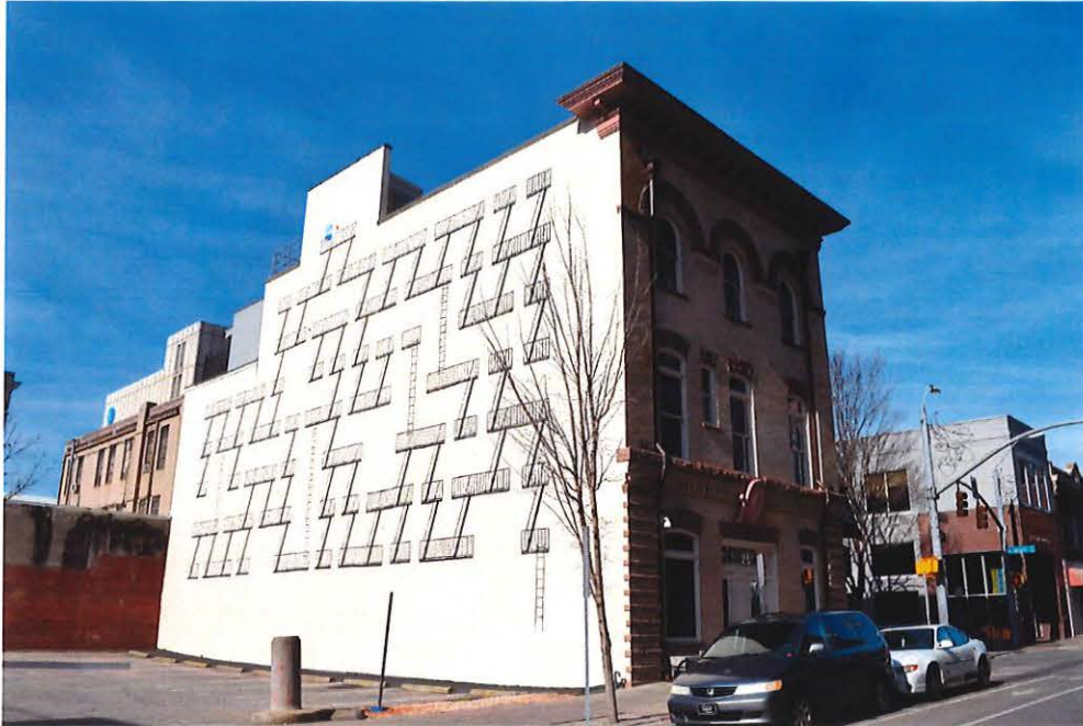
H. J. Brown Coffin House, south elevation, view NW
