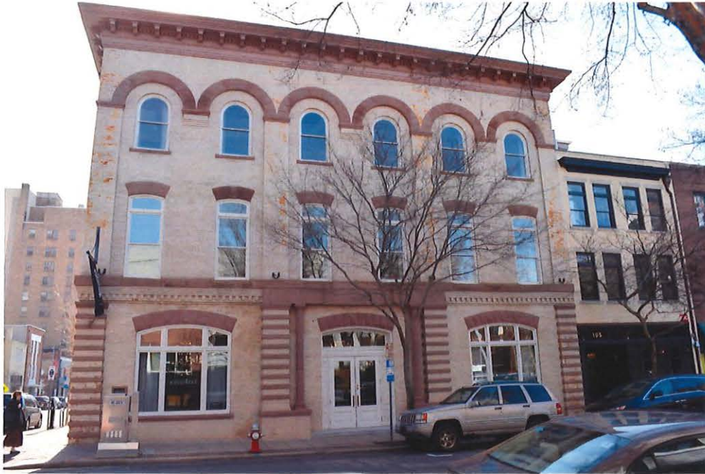
H. J. Brown Coffin Company, north elevation, view S
