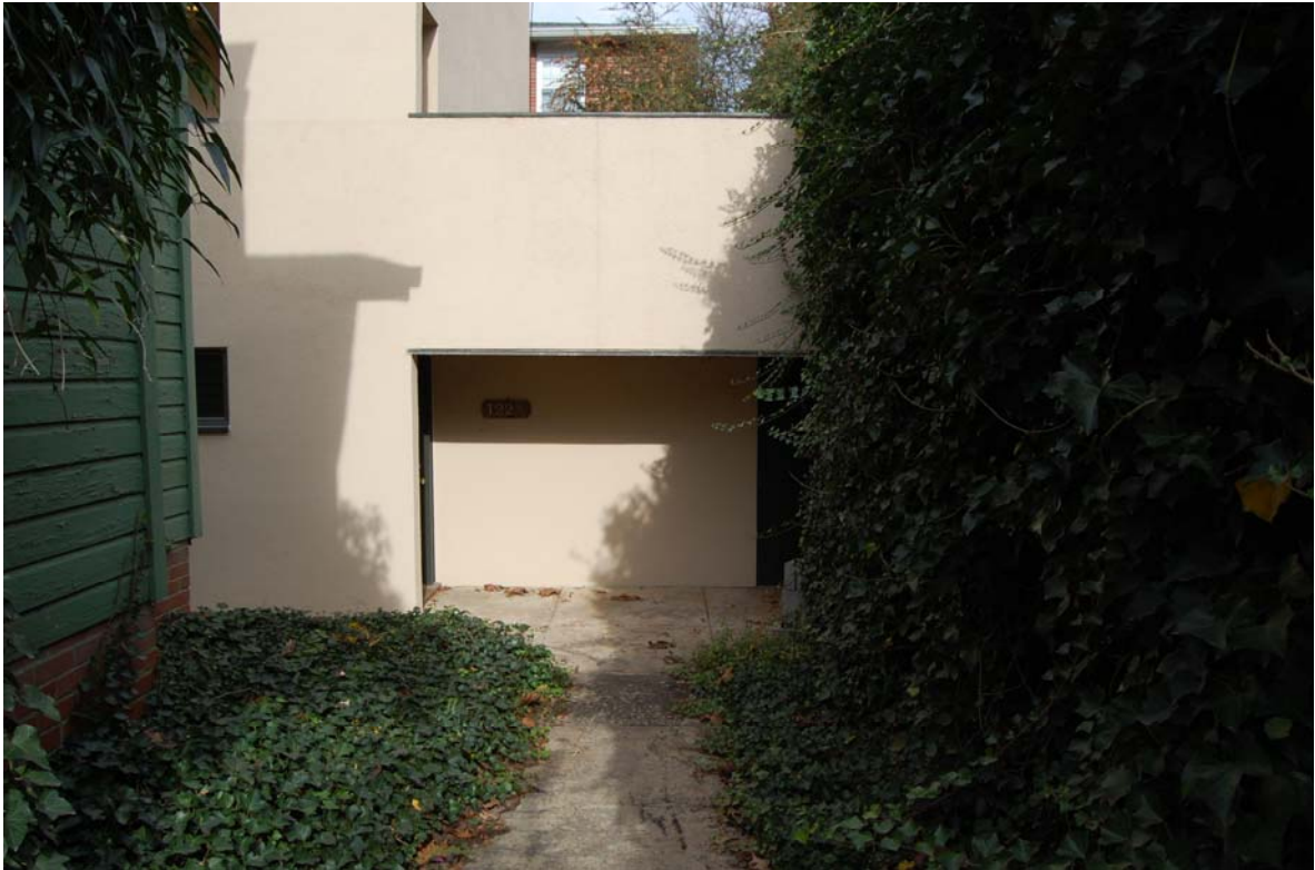
Entrance to basement level (north elevation)
