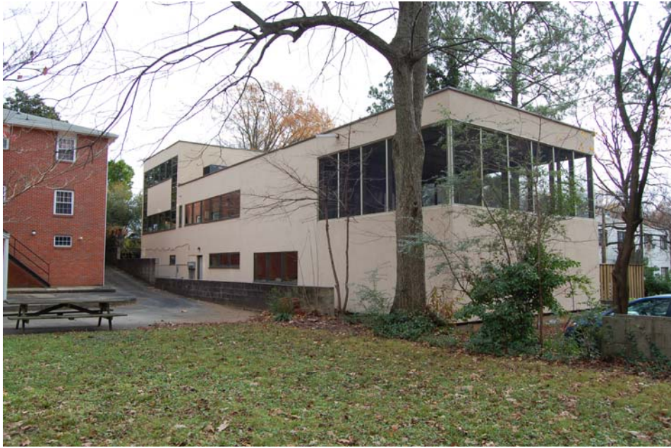
Façade (south and west elevations)
