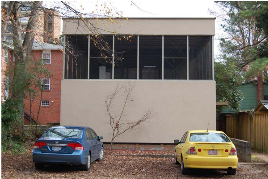
Façade (west elevation)
