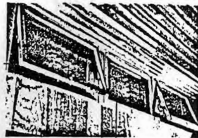
Ceiling vents let out heated air
