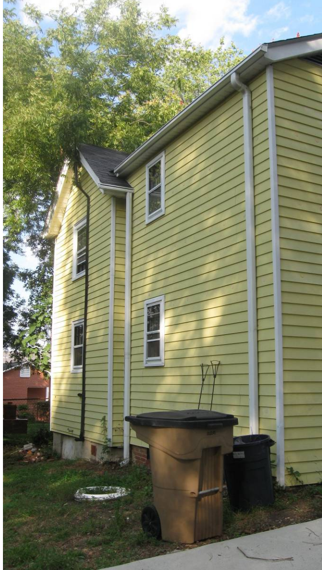
West (rear) facade
