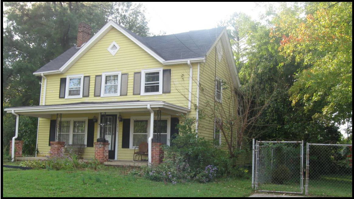
East and north façades
