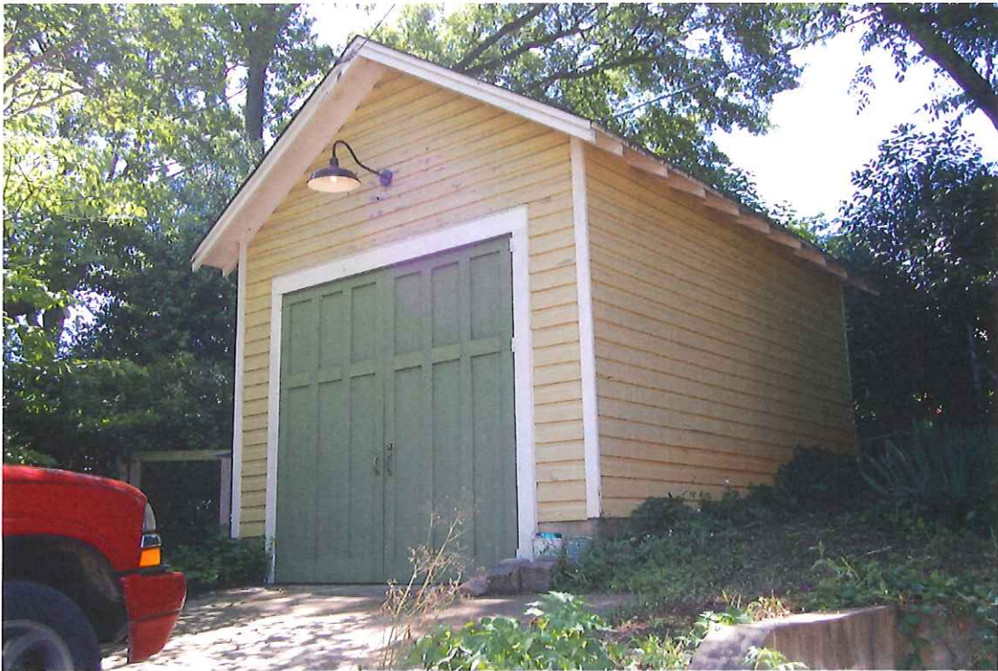
John and Belle Anderson House, 1201 Park Drive, garage, view SE
