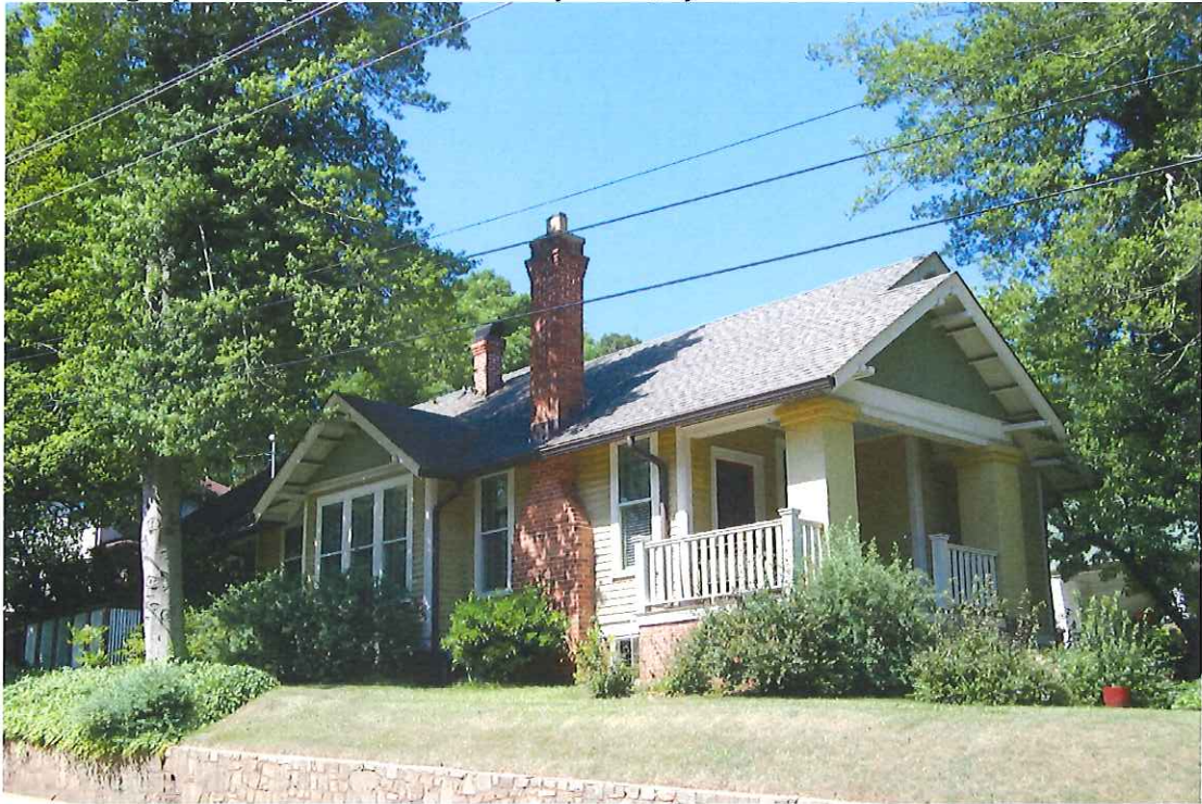
John and Belle Anderson House, 1201 Park Drive, facade & east elevation, view SW
