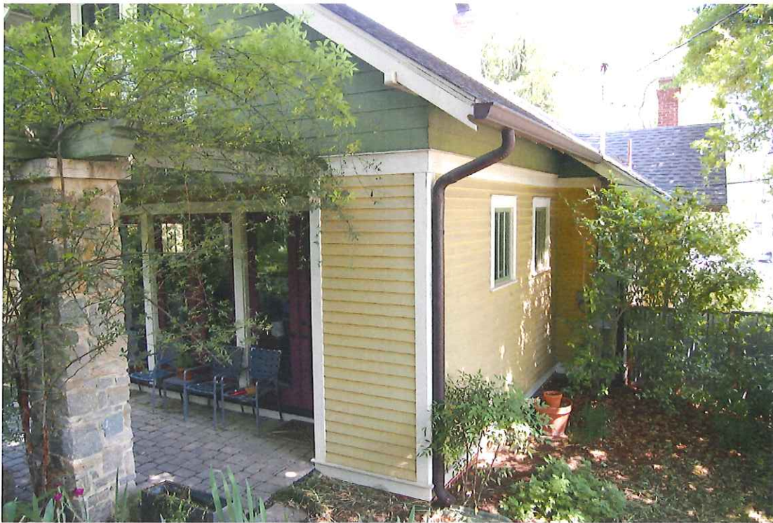
John and Belle Anderson House, 1201 Park Drive, rear and east elevations, showing juncture of addition and original dwelling, view NW
