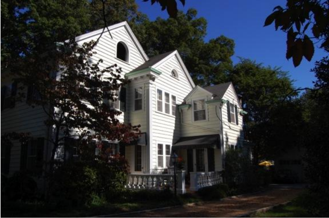
John E. Beaman House, 2120 White Oak Road, south elevation
