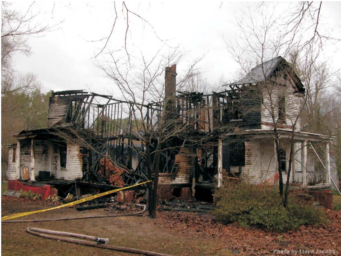
South and east elevations after fire.
