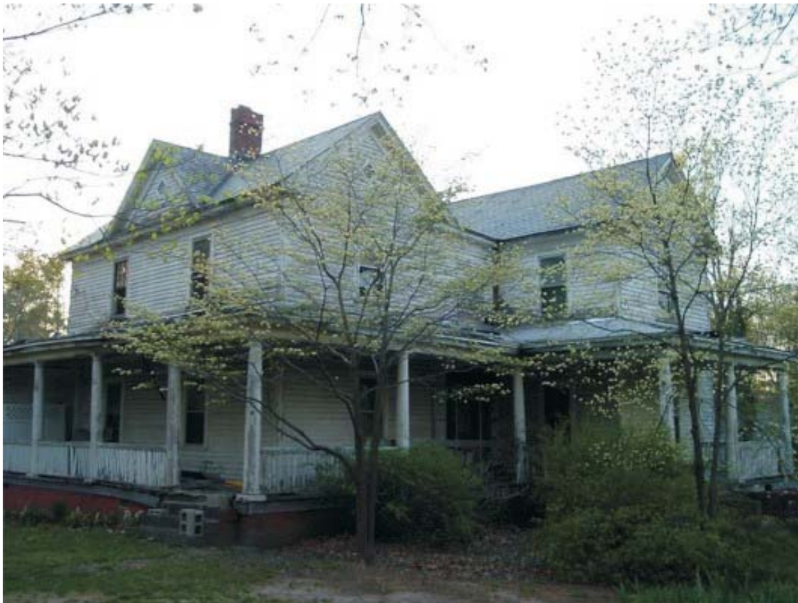
South and east elevations.
