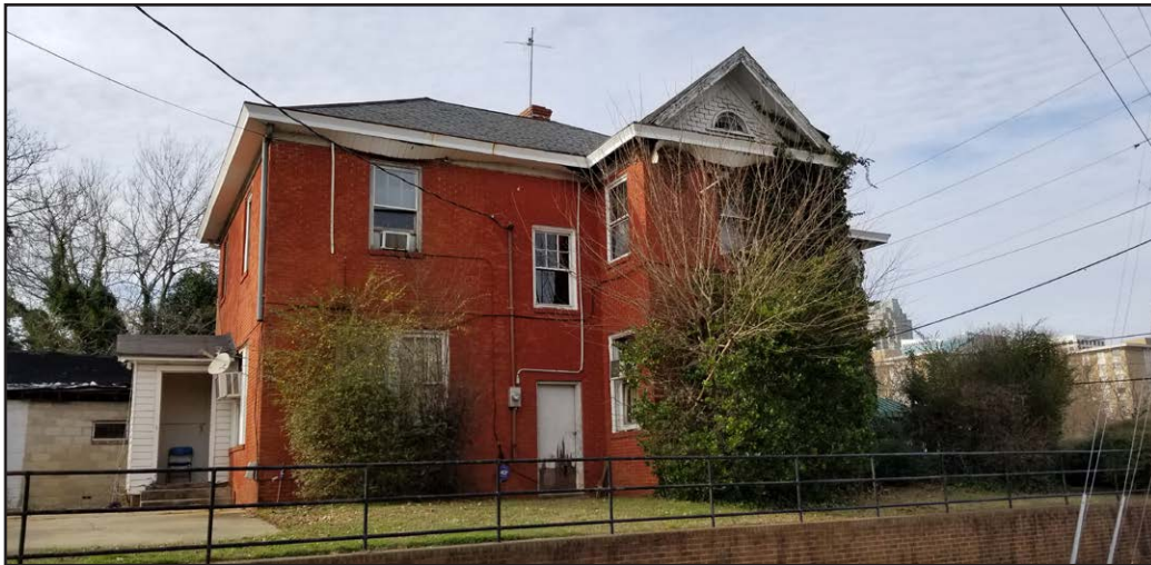
Plate 3.2: Capehart-Lightner House, Raleigh, North Carolina.
