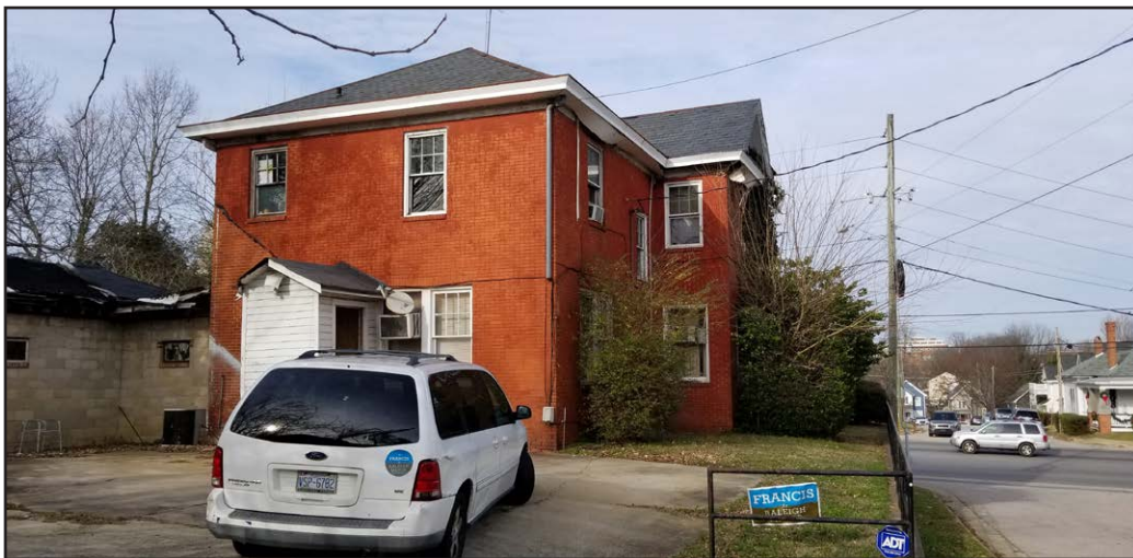
Plate 3.3: Capehart-Lightner House, Raleigh, North Carolina.
