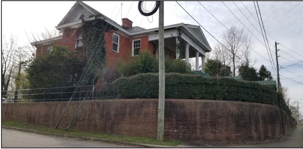
Plate 3.1: Capehart-Lightner House, Raleigh, North Carolina.
