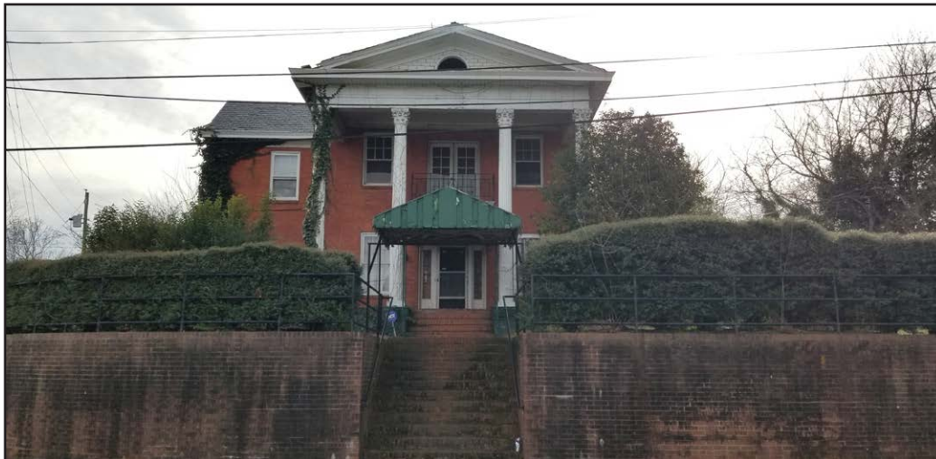
Plate 3.5: Capehart-Lightner House, Raleigh, North Carolina.
