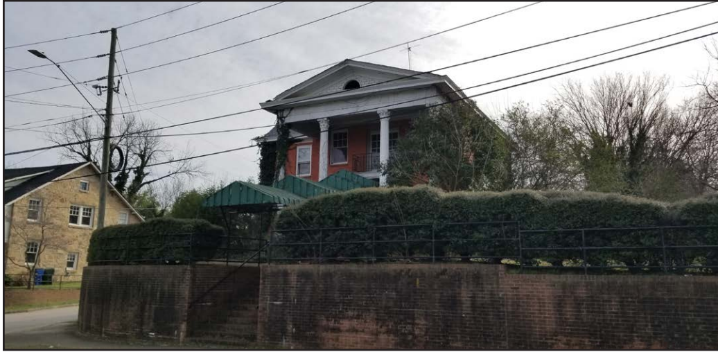
Plate 3.4: Capehart-Lightner House, Raleigh, North Carolina.
