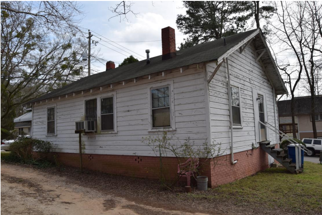
Lillie Stroud Rogers House, 616 Method Road, Raleigh, north and rear facades, view SE
