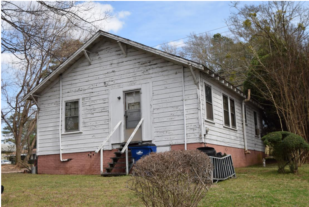
Lillie Stroud Rogers House, 616 Method Road, Raleigh, rear and south facades, view NE
