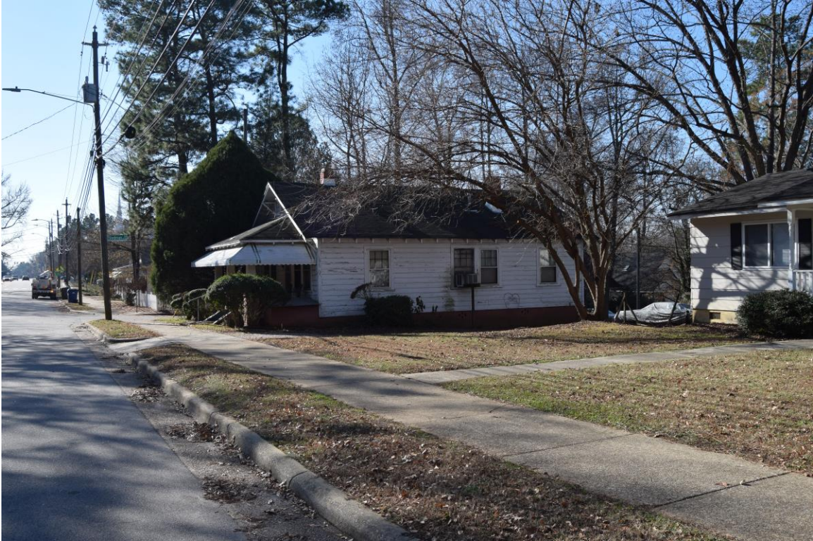
View of 616 Method Road and streetscape to the north, view SW
