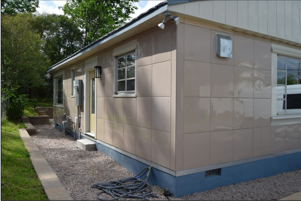
Photo 6. S side elevation, view NW.
