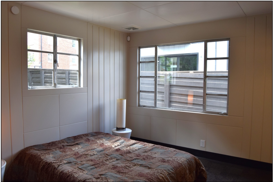
Photo 14. Interior at northwest bedroom, view NE.
