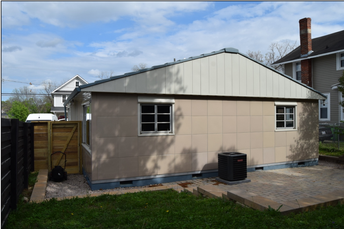
Photo 5. W (rear) elevation, view SE..
