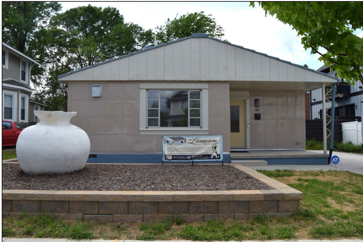
Photo 2. Façade, view W
