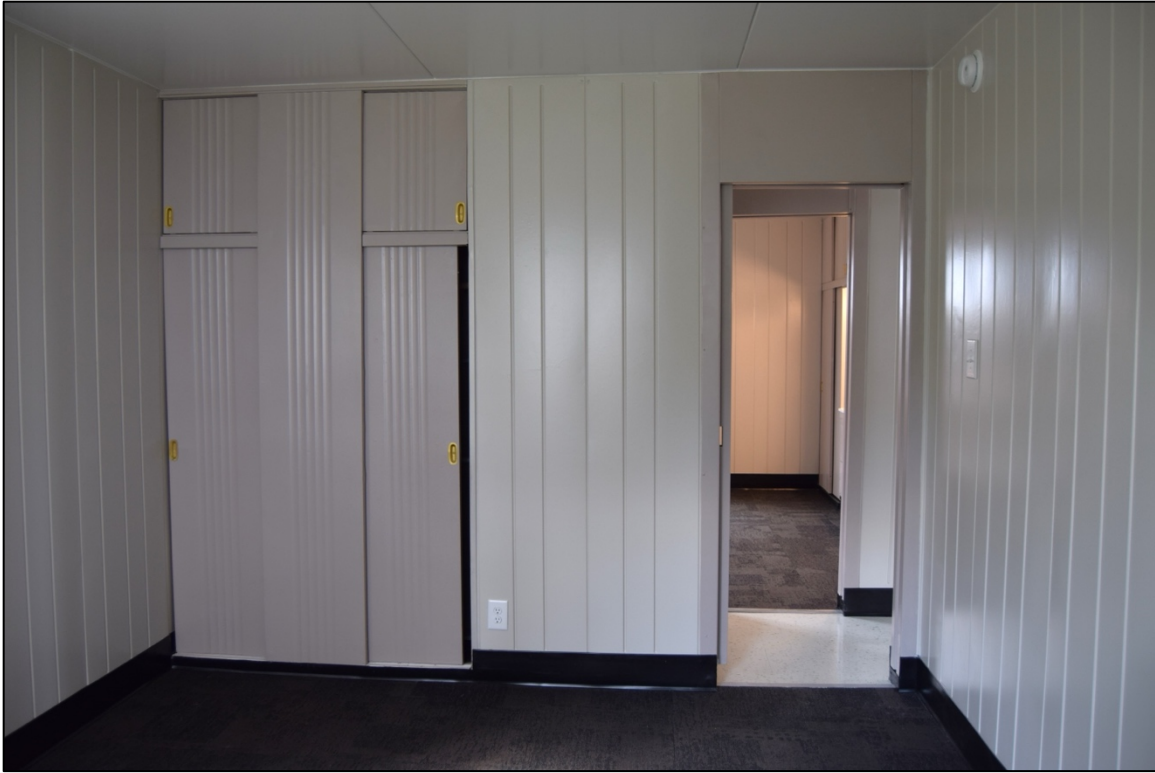
Photo 16. Interior at southwest bedroom, view N.
