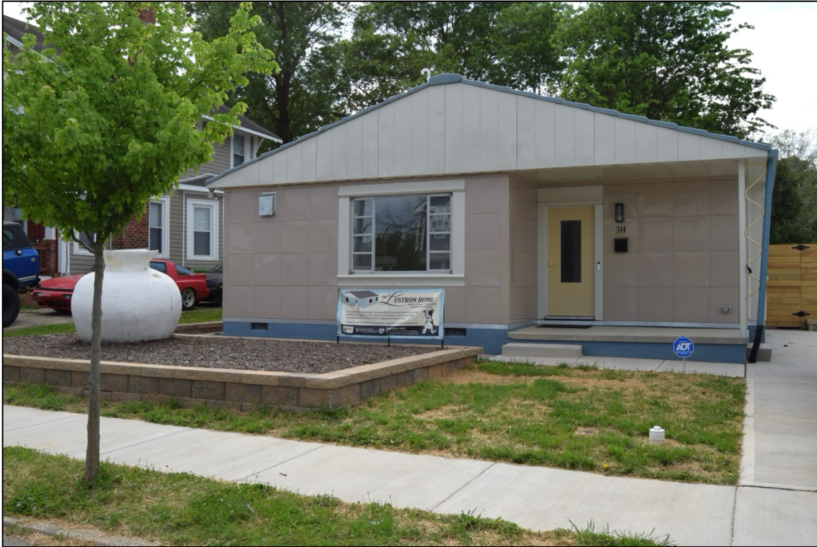
Photo 1. Overall view showing façade and front-yard planter, view SW.
