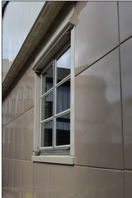
Photo 7. Bathroom window at S side elevation, view NW.
