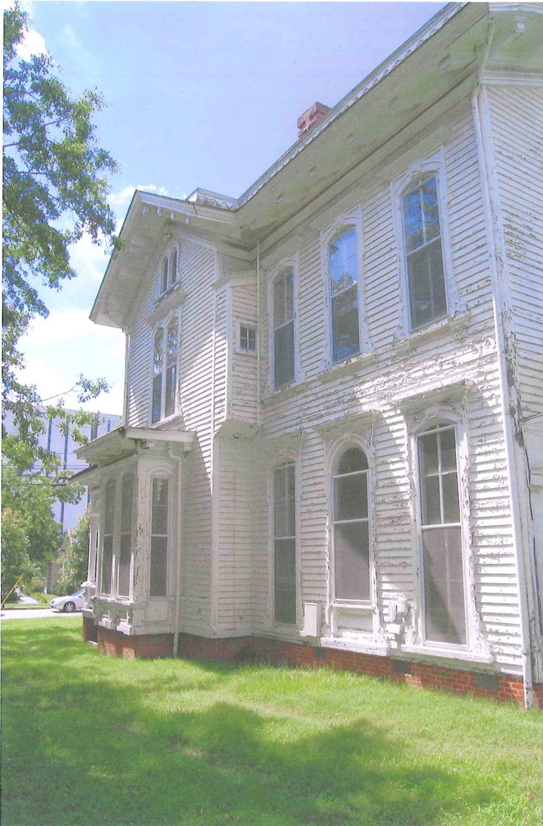
Merrimon-Wynne House, 500 N. Blount Street, view NW
