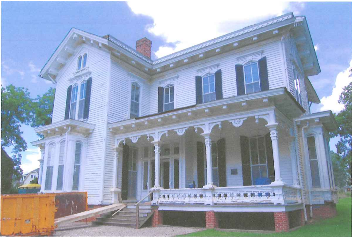
Merrimon-Wynne House, 500 N. Blount Street, view NE
