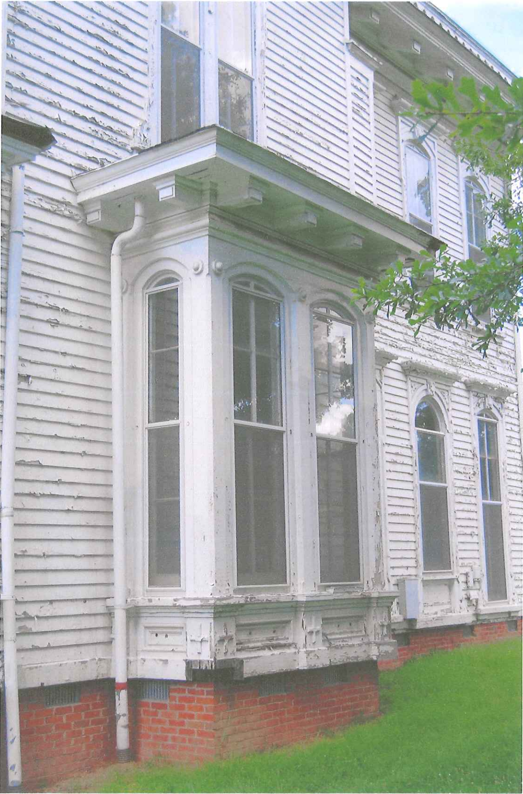
Merrimon-Wynne House, 500 N. Blount Street, view NE
