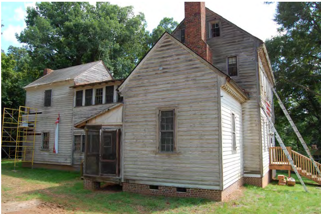
North (side) elevation, view SE
