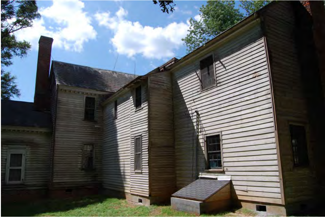
South (side) elevation, view NW
