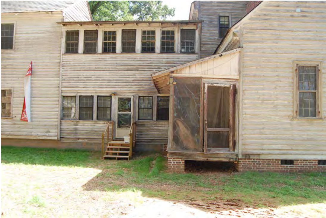
North (side) elevation, view S
