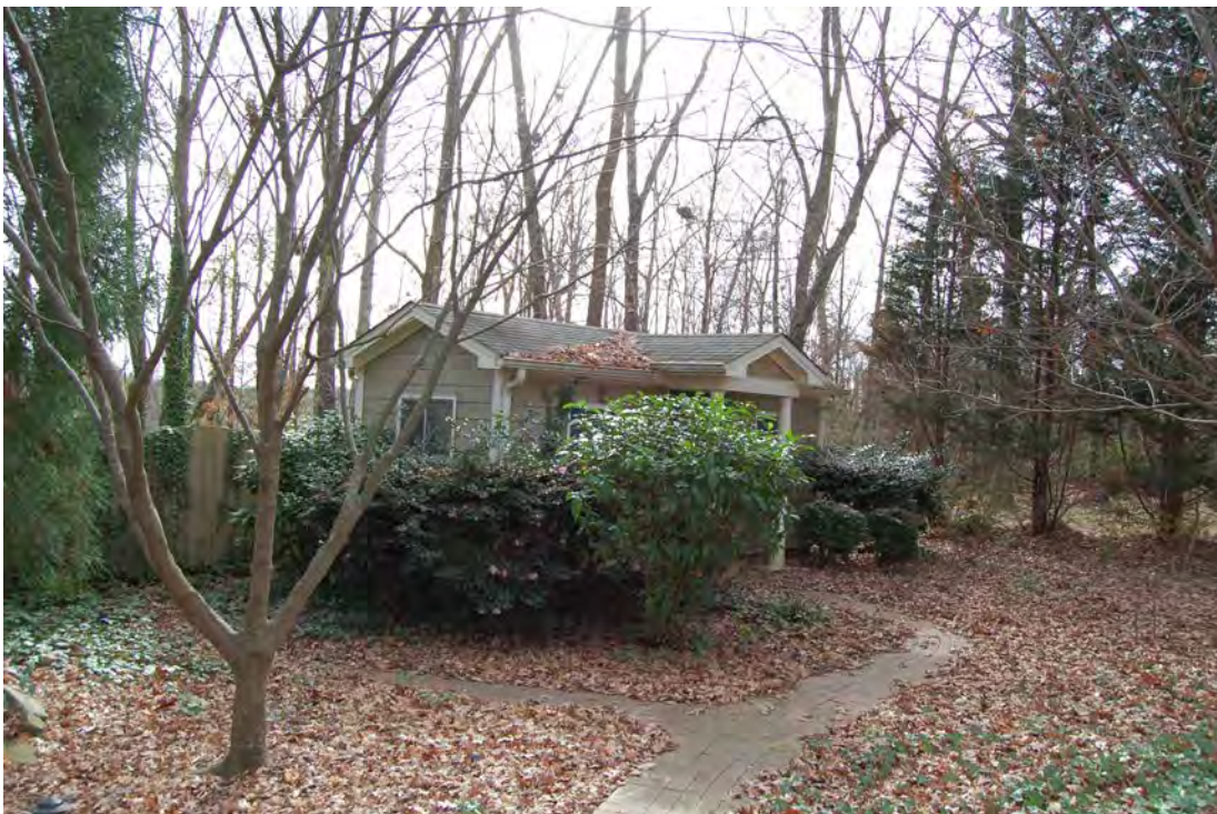
Outbuilding, view SE
