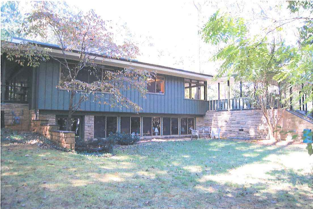
Owen and Dorothy Smith House, 122 Perquimans Drive, Raleigh, Wake County East elevation, view NW
