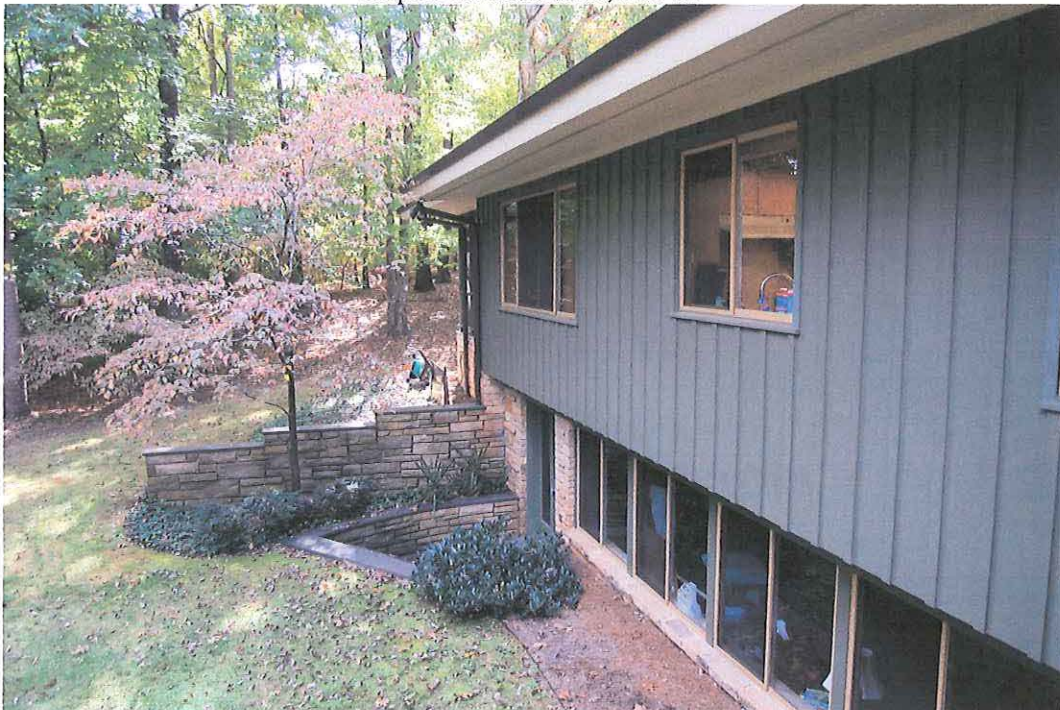
Owen and Dorothy Smith House, 122 Perquimans Drive, Raleigh, Wake County East elevation, view SW
