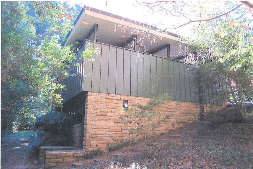
Owen and Dorothy Smith House, 122 Perquimans Drive, Raleigh, Wake County Carport north elevation, view SW
