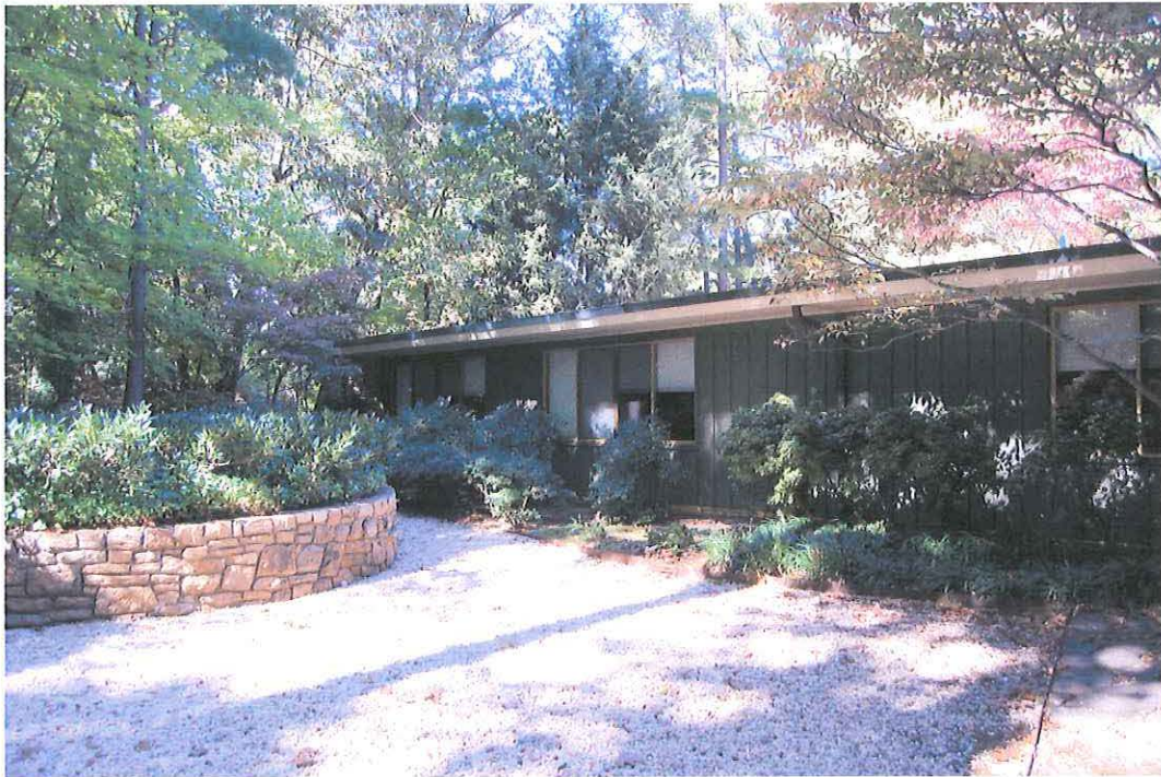
Owen and Dorothy Smith House, 122 Perquimans Drive, Raleigh, Wake County Rear elevation of front wing, backyard landscaping. View NW.
