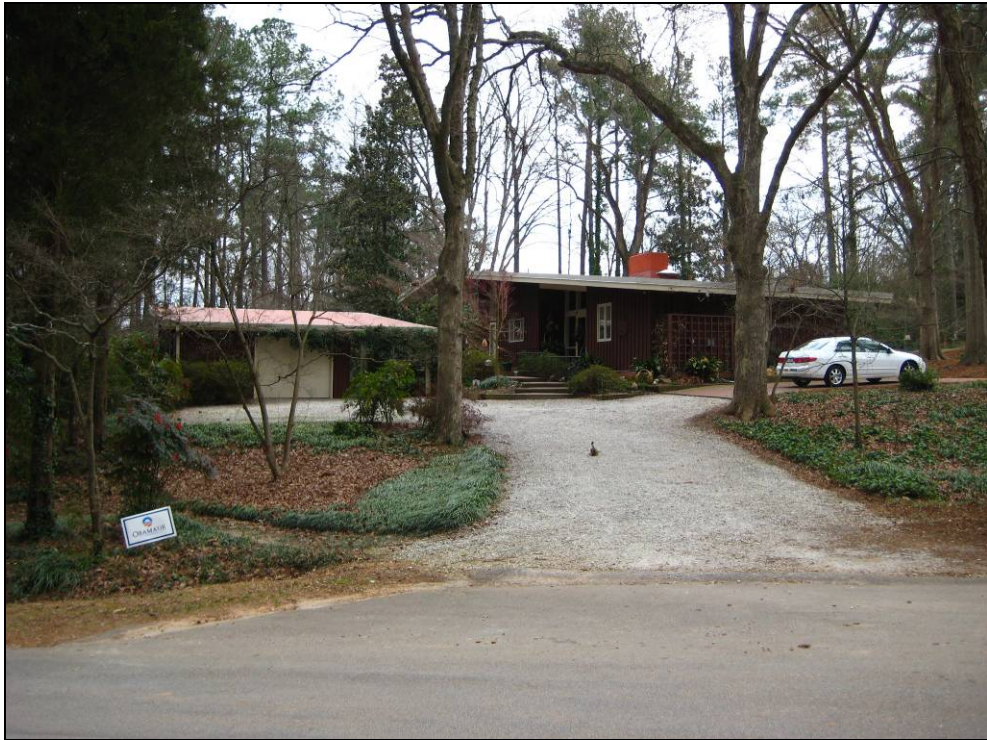
Façade View (NW corner)
