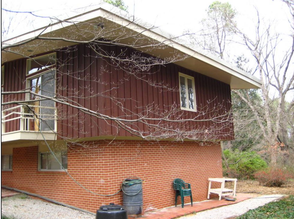
SE corner (view of rear and east/side elevation)
