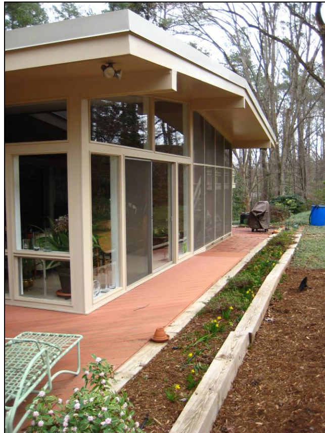
Eave detail on rear/SW elevation
