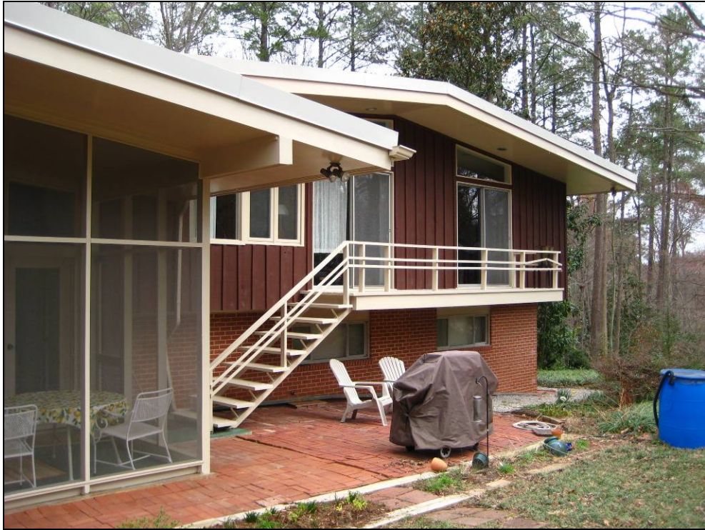
Detail of Rear/SW elevation (rear deck and stair)
