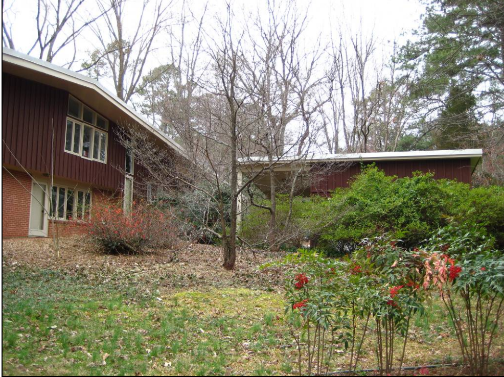
Garage (Rear/SE elevation)
