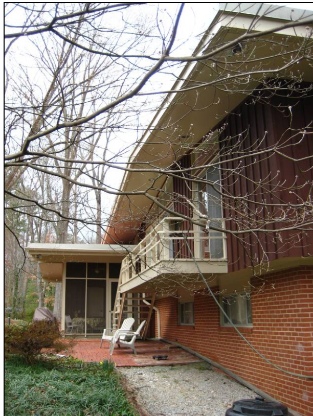
Eave and rear deck/stair detail (SE corner)
