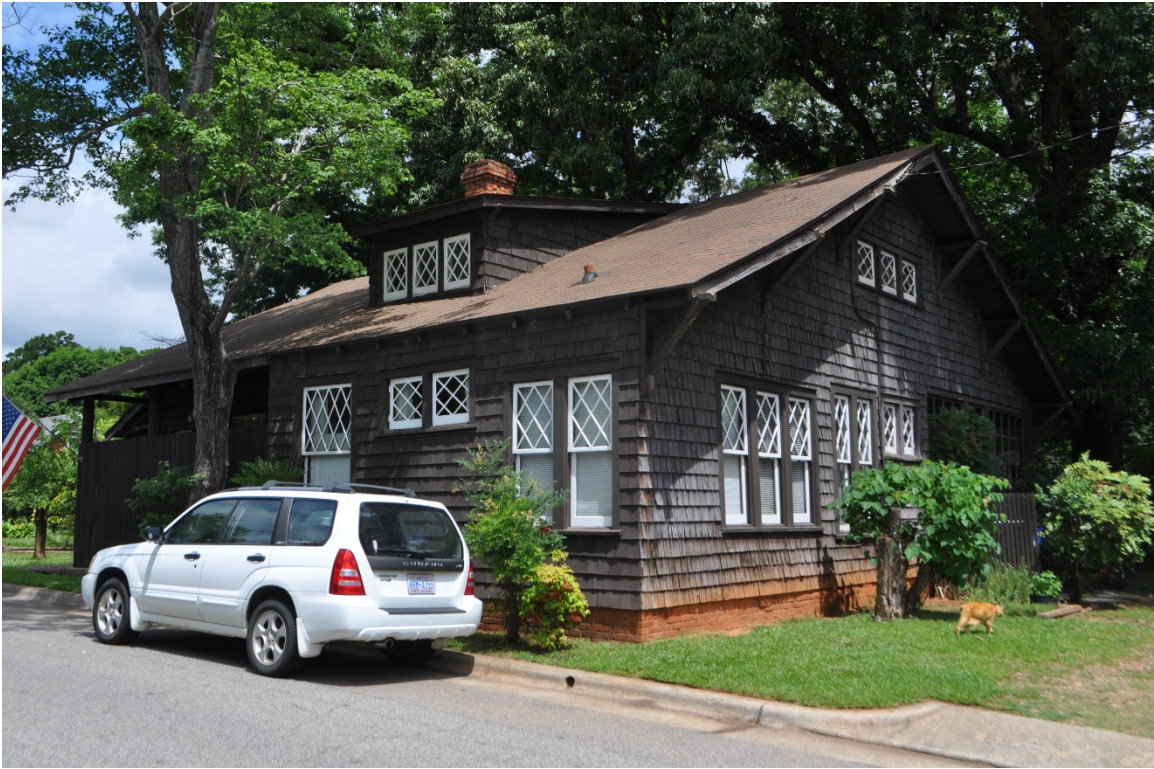
Plate 3: South and east elevations of the house.
