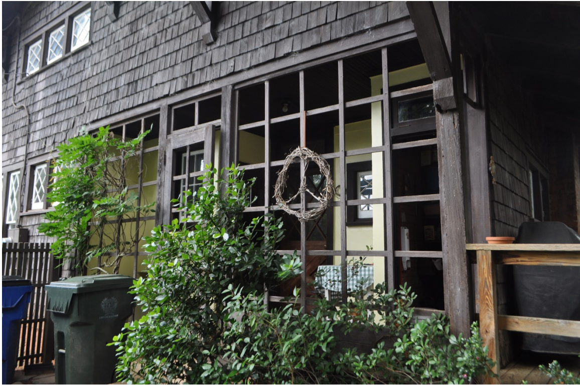
Plate 9: Detail view of the inset porch on the east elevation.
