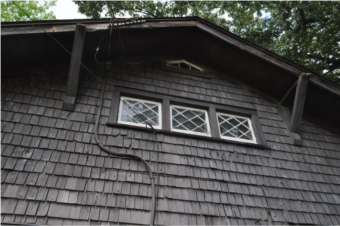
Plate 13: Detail view of the typical casement windows found throughout the house.
