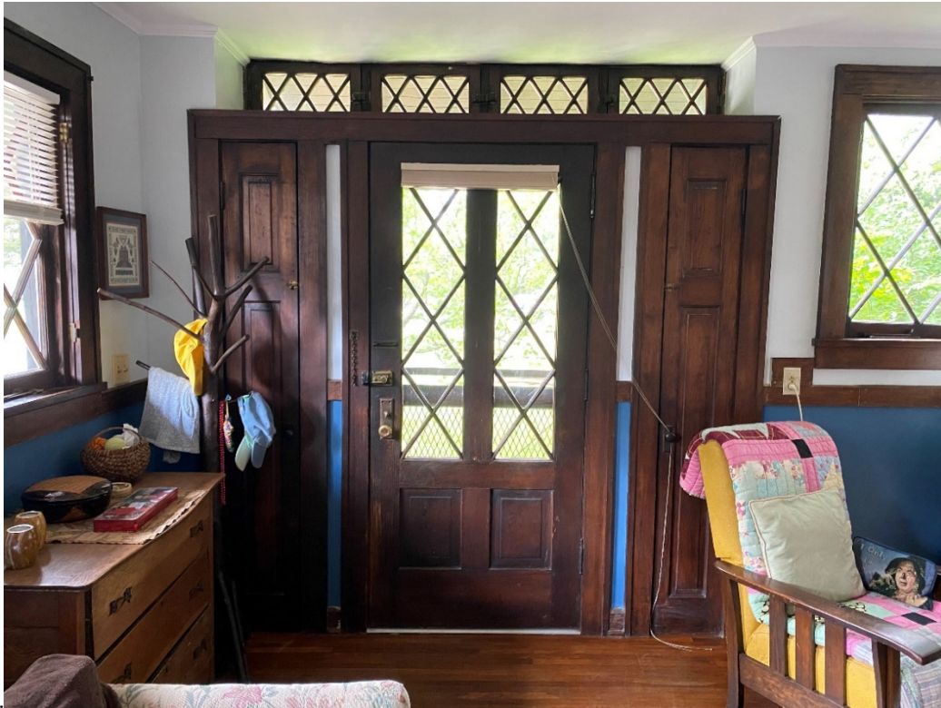
Plate 17: Detail view of the front door with its flanking, built-in closets.
