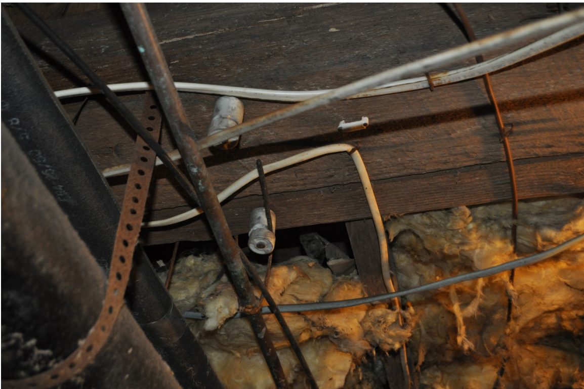
Plate 26: Detail view of the original knob and tube wiring system.
