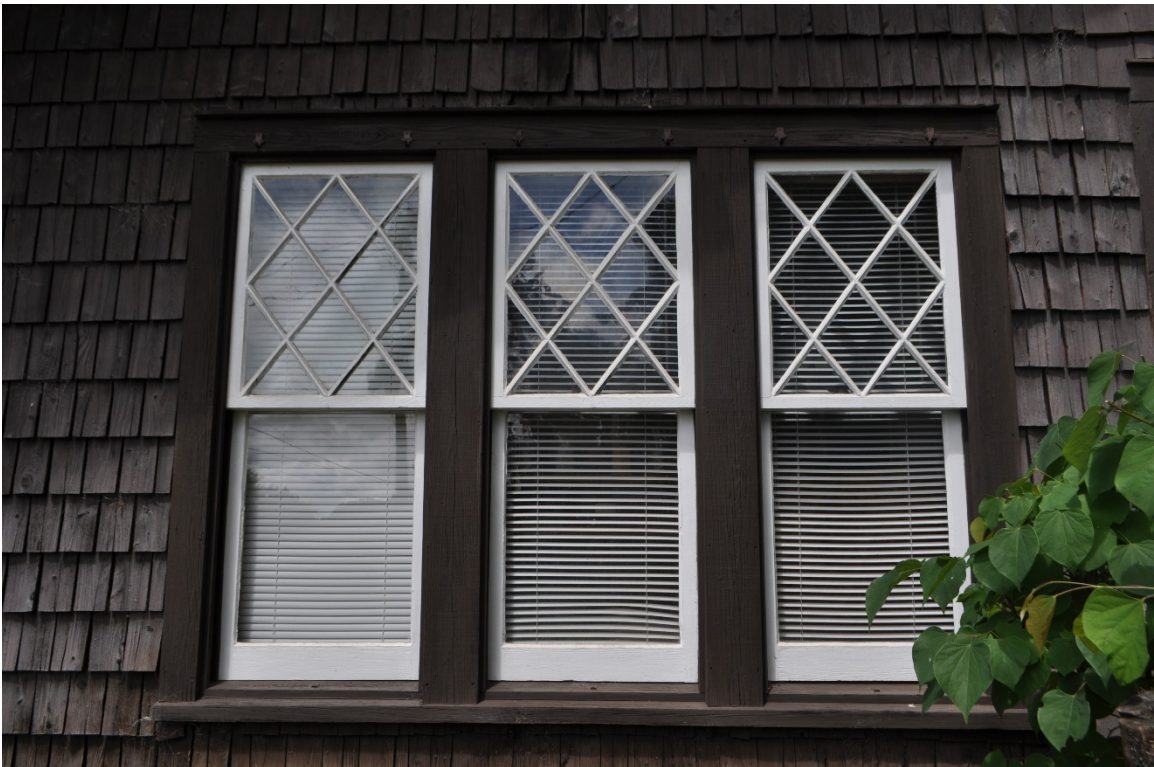
Plate 12: Detail view of typical window sashes found throughout the house.
