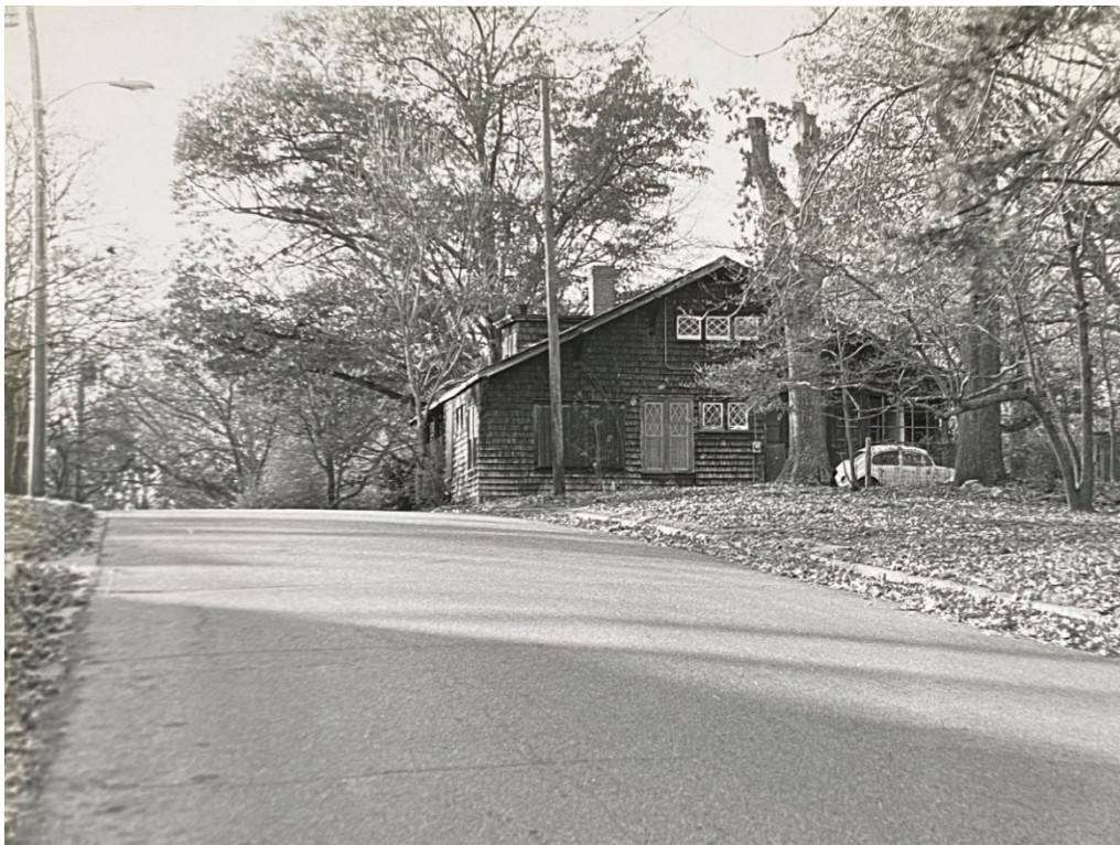
Figure 12: View of the east elevation of Pitysmont in the 1980s (Courtesy of Tony and Jenny McGrail).
