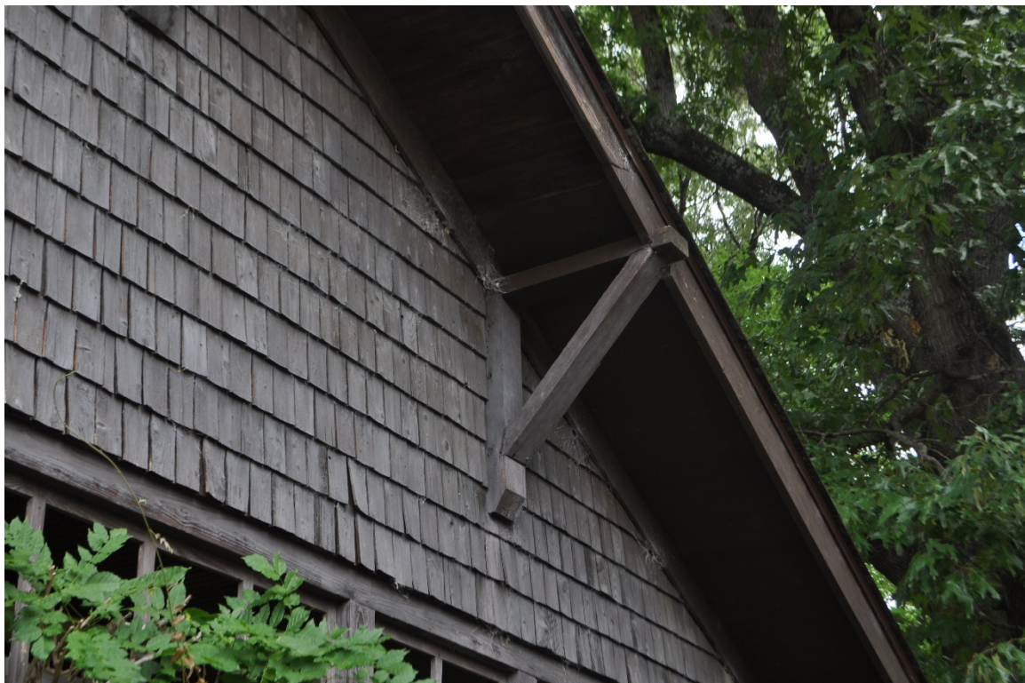
Plate 14: Detail view of the decorative wood brackets in the eaves of the east and west elevations.
