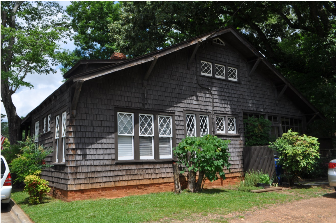
Plate 4: East elevation of the house.
