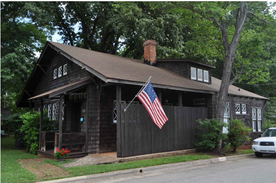
Plate 2: Primary (west) and south elevations of the house.
