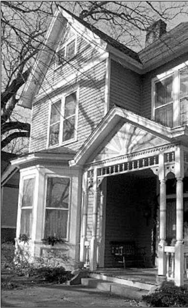
Turned spindles and columns, pierced brackets, and a radiating pattern of flush boards in the porch gable of this clapboard house illustrate the versatility of wood for detailing.
