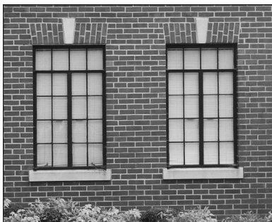
Rolled steel casement windows are hinged vertically and are distinctive features found on many buildings from the 1920s and 30s.
