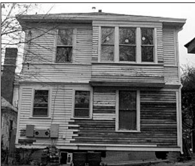
During rehabilitation, replacement siding to match the original siding was carefully incorporated on this rear facade before repainting.
