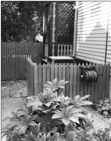
This mechanical unit was installed on a rear side facade and further screened from view by a low, wooden picket fence and foundation plantings.
