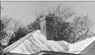
Standing-seam metal roofs must be kept painted, or they will begin to corrode.
