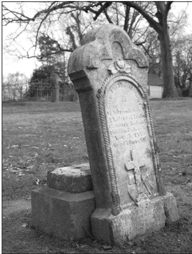
This gravestone at O'Rourke Cemetery is detached from its base. Reinstalling it could cause more damage if not overseen by an experienced stone conservator.
