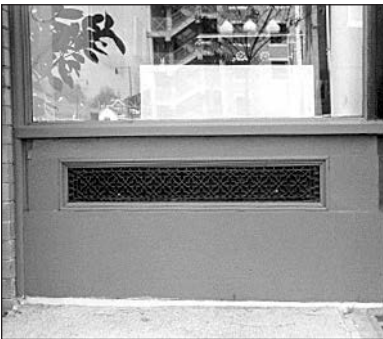
The cast-iron grille recessed within this storefront bulkhead panel is both decorative and functional.
