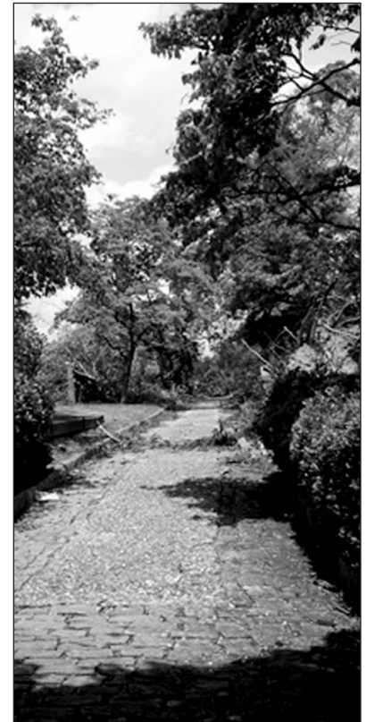
Surrounded by mature trees and shrubs, the central circulation path through City Cemetery is paved with brick pavers with a stone median and edged by stone curbs.
