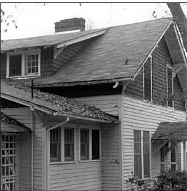
A missing downspout from the main gable and a large collection of fallen leaves will accelerate the deterioration of the shingles on the rear gable of this roof.
