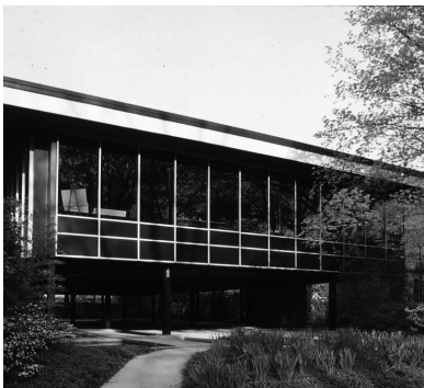
The curtain wall facade of this Raleigh landmark is characteristic of many mid-century modern office buildings which embraced large spans of non-loadbearing glass walls.
