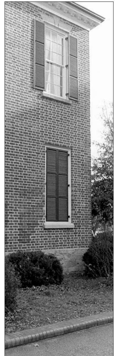
Louvered shutters provide a traditional means of shading the sun's heat from the interior of a structure while providing ventilation.
