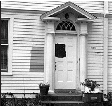
In selecting new paint colors for this residence, test areas of proposed colors were applied to the facade for viewing.
