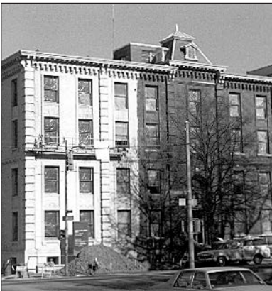
Layers of paint were successfully chemically stripped from the Labor Building's facades during a major rehabilitation.
