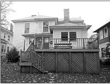
Wooden decks like these, located on rear facades with simple balustrades, skirt boards, and lattice infill panels between supports, are appropriate in the historic districts.
