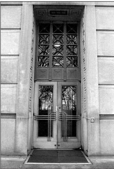
The architectural significance of the decorative metal work on the front entrances to the Justice Building warranted automating this pair of steel doors rather than replacing them to meet accessibility requirements.
