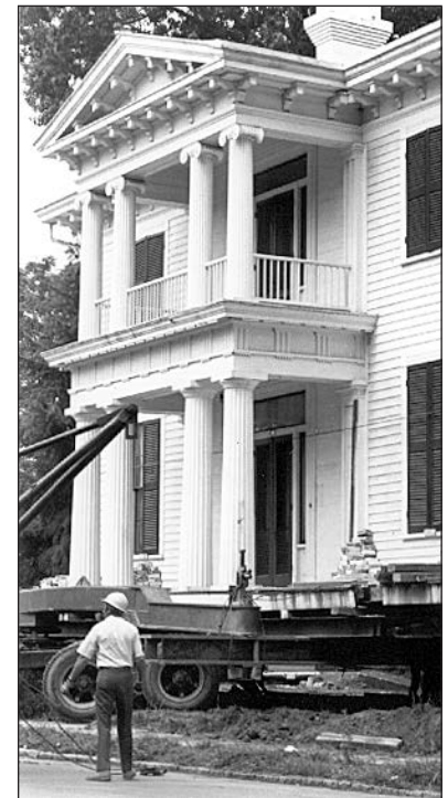
Even the two story portico of the Lewis-Smith House remained attached during its relocation.
