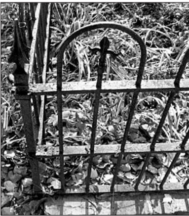
The paint film on this cast-iron fence is failing because of corrosion. All rust must be removed before repainting.
