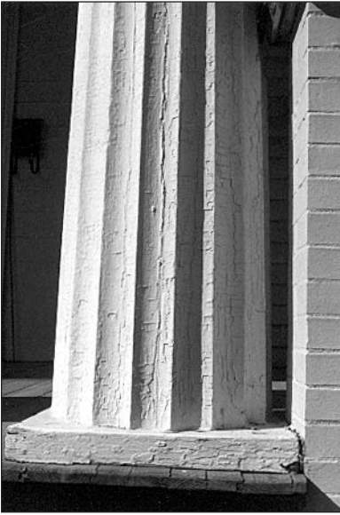
When multiple layers of paint begin to check and alligator, as this column's surface has, they must be scraped and sanded down to the first sound paint film layer before repainting.
