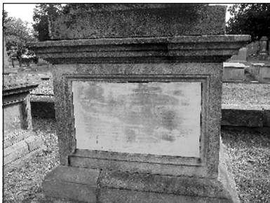
Unfortunately, the inscription on the marble face of this historic grave marker was damaged when it was cleaned with bleach and it is now illegible. Rather than falsify the stone by re-inscribing it, a new inscribed plaque could be placed nearby on a separate base.
