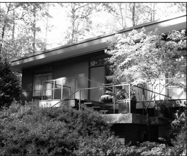
The raised front entrance to this modernist home continues across the front of the house as a narrow cantilevered deck partially sheltered by the roof overhang.
