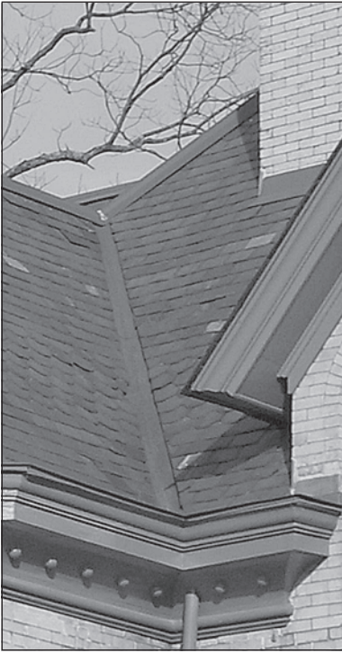
This well-maintained slate roof includes valleys and crestings that have a sound paint film protecting them from corrosion.
