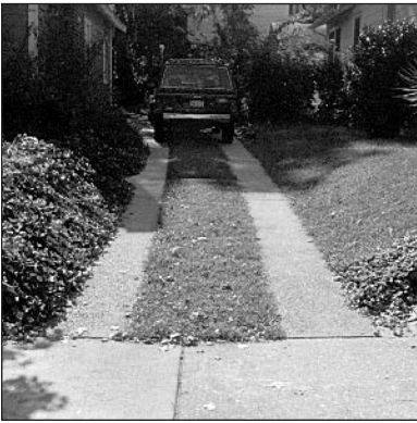
Simple driveways consisting of concrete or gravel runners with a grassy median are typical in the early residential historic districts.
