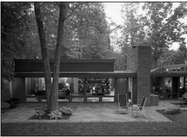
The large expanses of glass framed in wood in this landmark early modernist house create a strong connection between the interior and the backyard patio. The massive brick chimney wall visually anchors the glazed exterior walls on either side.
