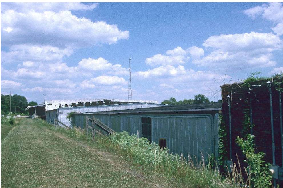
Rear view from railroad right-of-way
