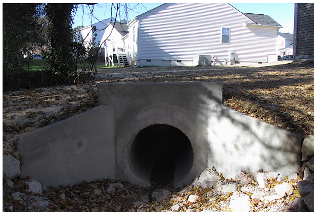
A stormwater pipe that's extended to reduce erosion on a Toccopola St. property.
