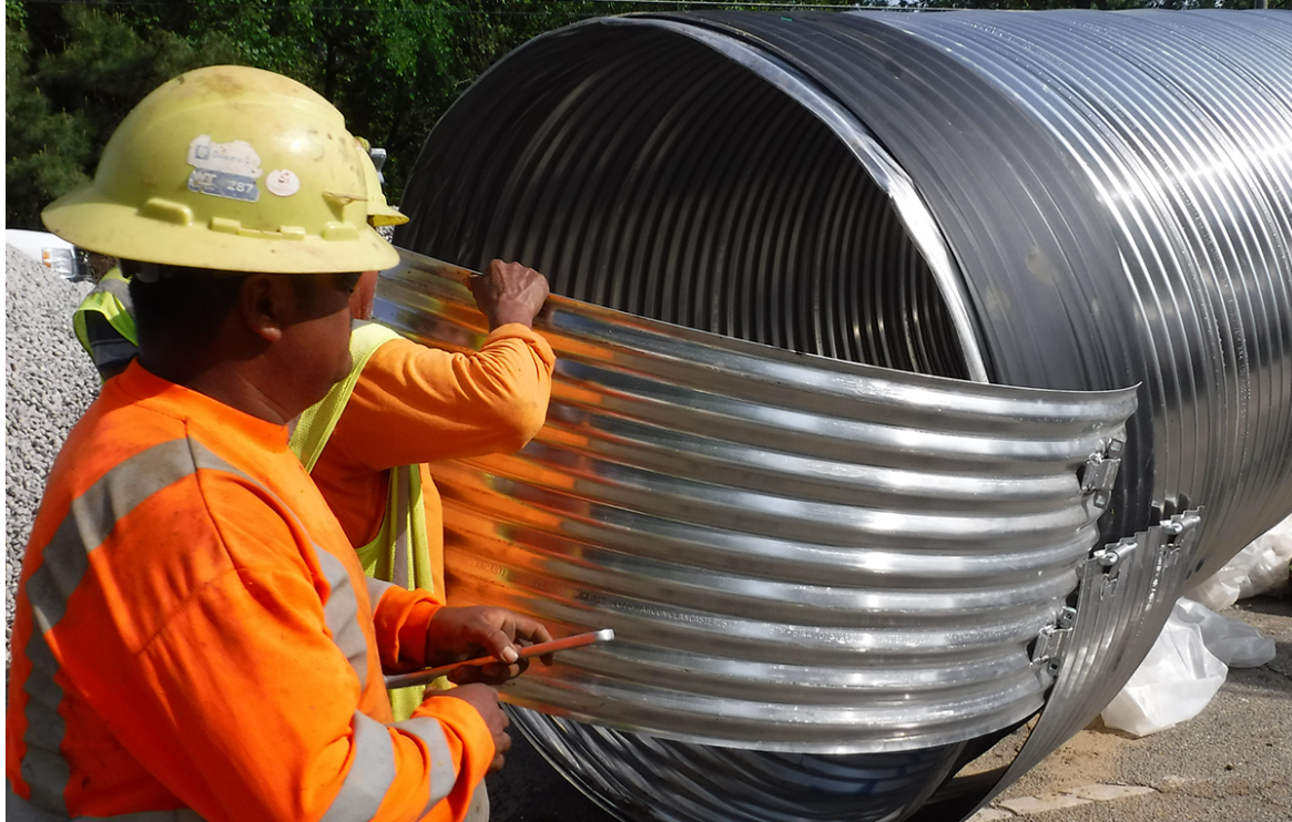
Crews installing a new stormwater pipe on Lake Wheeler Rd.
