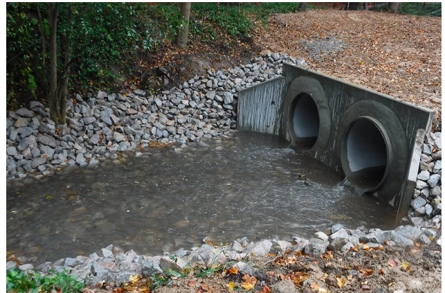
New stormwater pipes on Clark Ave. that will carry rainwater through the drainage system during a storm.
