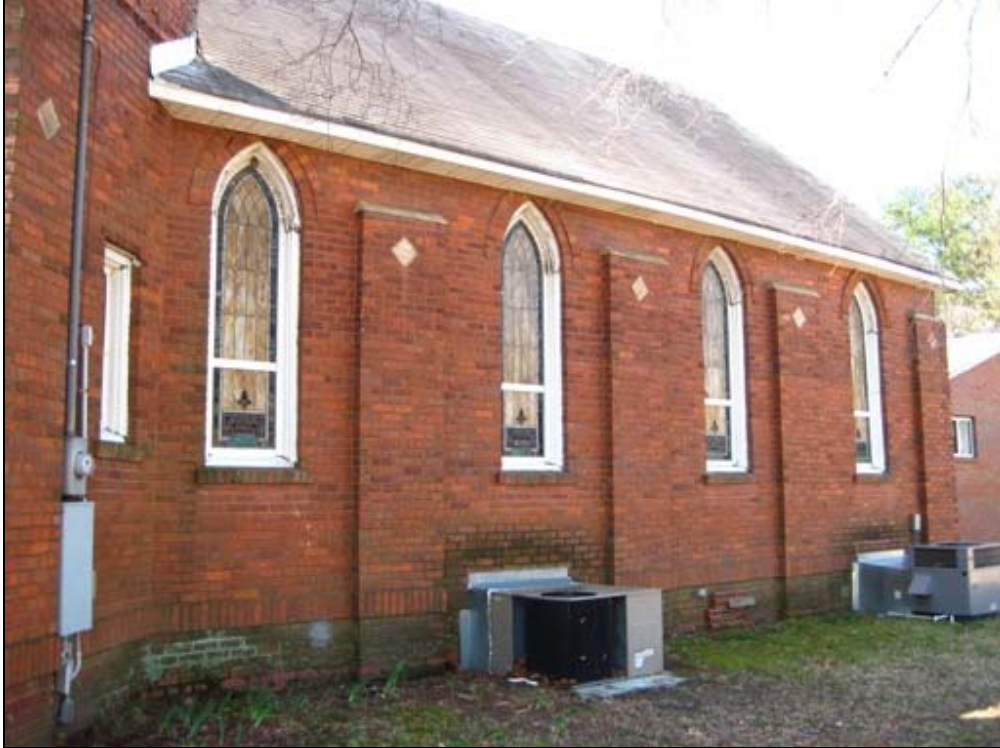
Buttresses (north elevation)
