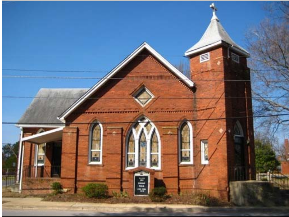
Façade/East Elevation detail
