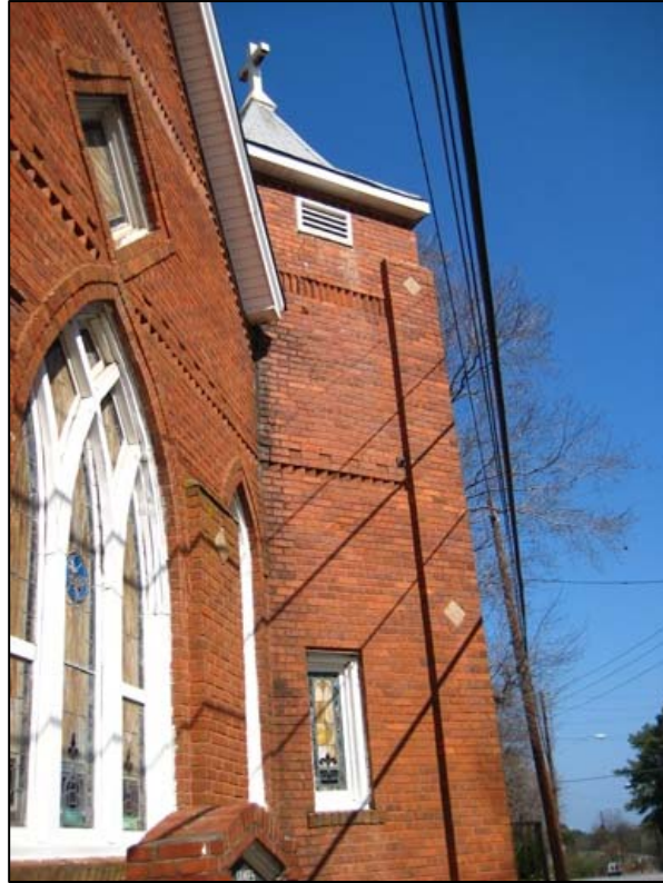
Corbelled brickwork on facade
