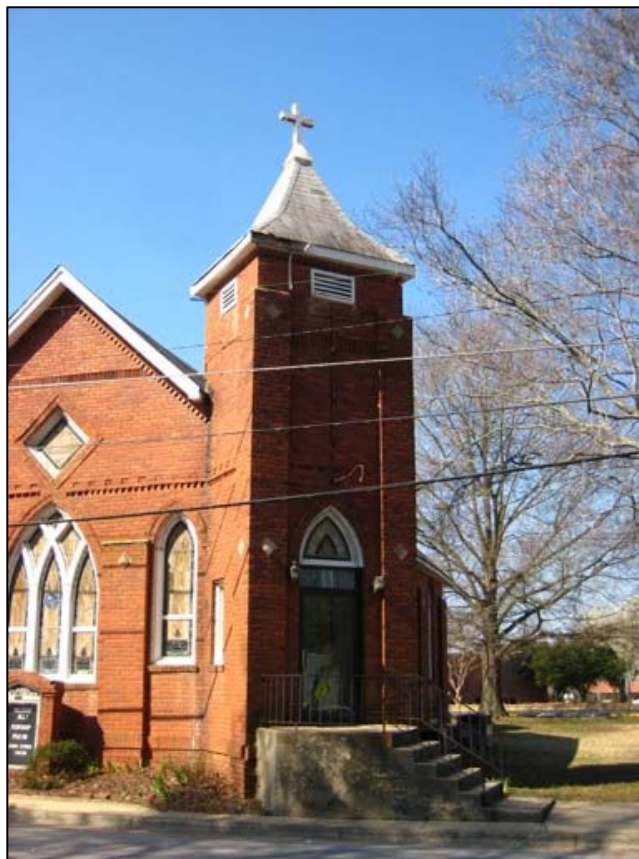
Steeple Tower (northeast corner)
