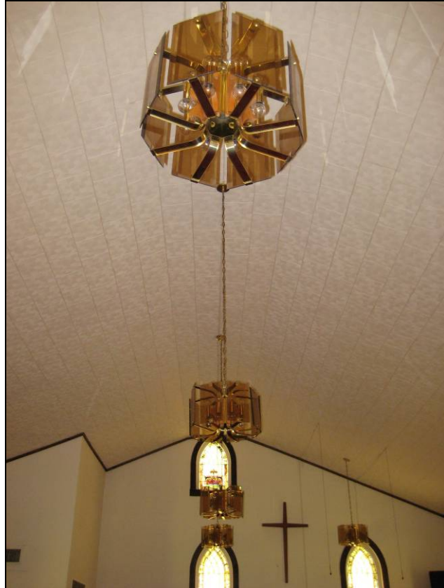
Detail of Ceiling and Light Fixtures (c.1970)
