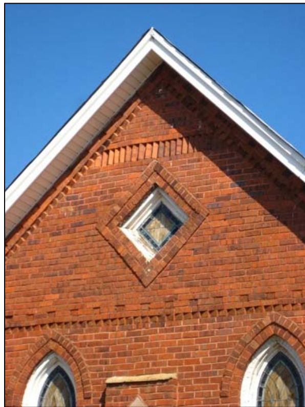
Corbelled brickwork detail (south gable end)
