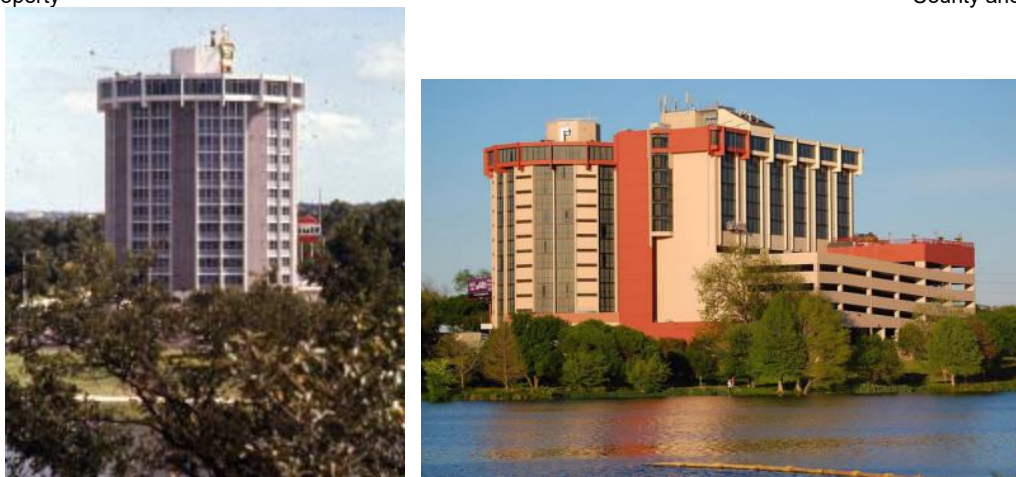
Figure 6: Austin Town Lake Holiday Inn, the original 1964 design featured a focus on the building's cylindrical and vertical design (left). Today, the building features large additions and alterations to the building's exterior cladding and fenestration (right). 16
