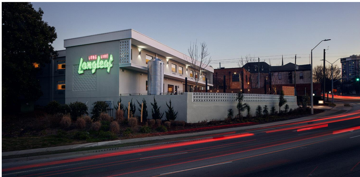
Figure 3: View of the 1964 Days Inn at 300 N. Dawson Street, which reopened ca. 2019 as the Longleaf Hotel and Lounge. The renovation uncovered some previously hidden mid-century details (source: https://www.thelongleafhotel.com/gallery )
