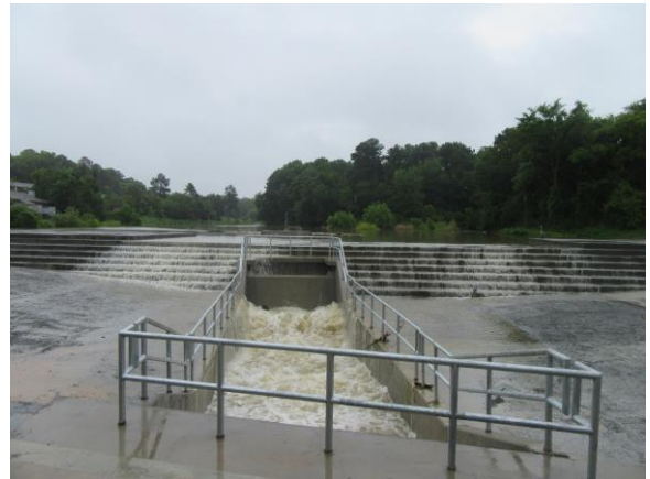
The tiered, reinforced concrete structure at Brockton Drive Lake during Tropical Storm Elsa in July 2021.
