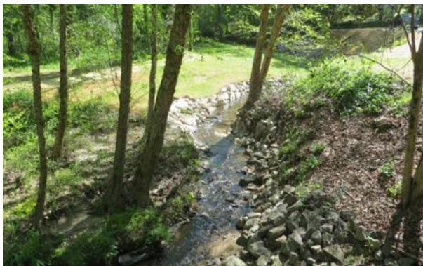
The stream stabilization on Gainsborough Drive after construction.
