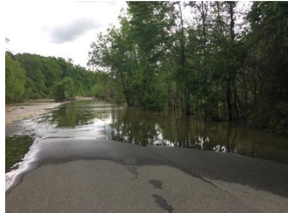
Flooding on Rose Lane in Raleigh.
