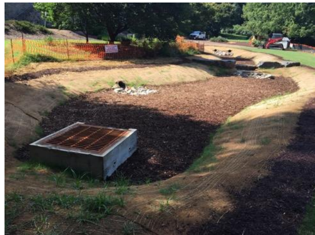
The bioretention area under construction at the Rose Garden in Raleigh.
