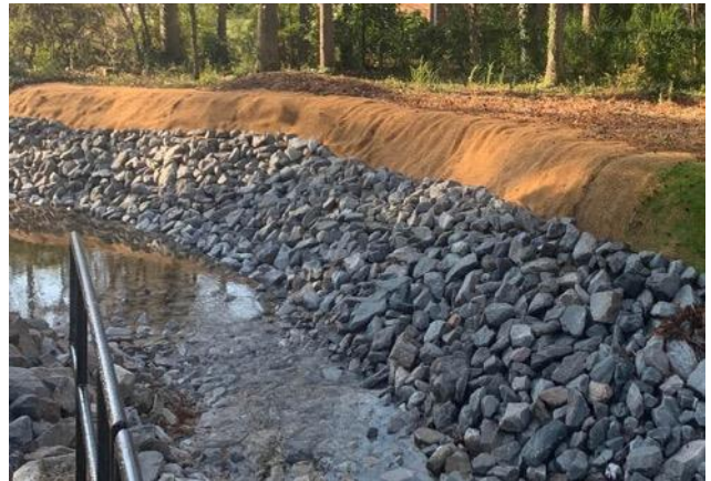
A repaired streambank along Swift Drive in Raleigh.
