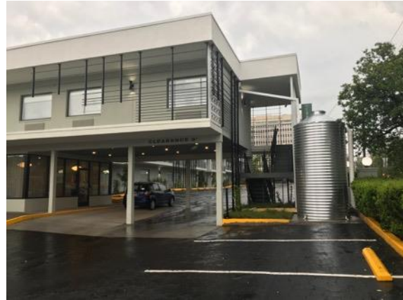
One of six cisterns at the Longleaf Hotel in downtown Raleigh. The system can collect about 5,500 gallons of water when it rains.
