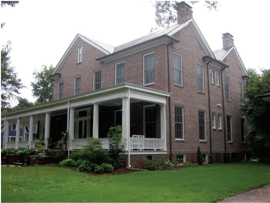
1 Exterior NW Corner
