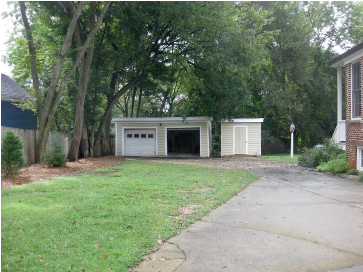
8 Shed and Garage
