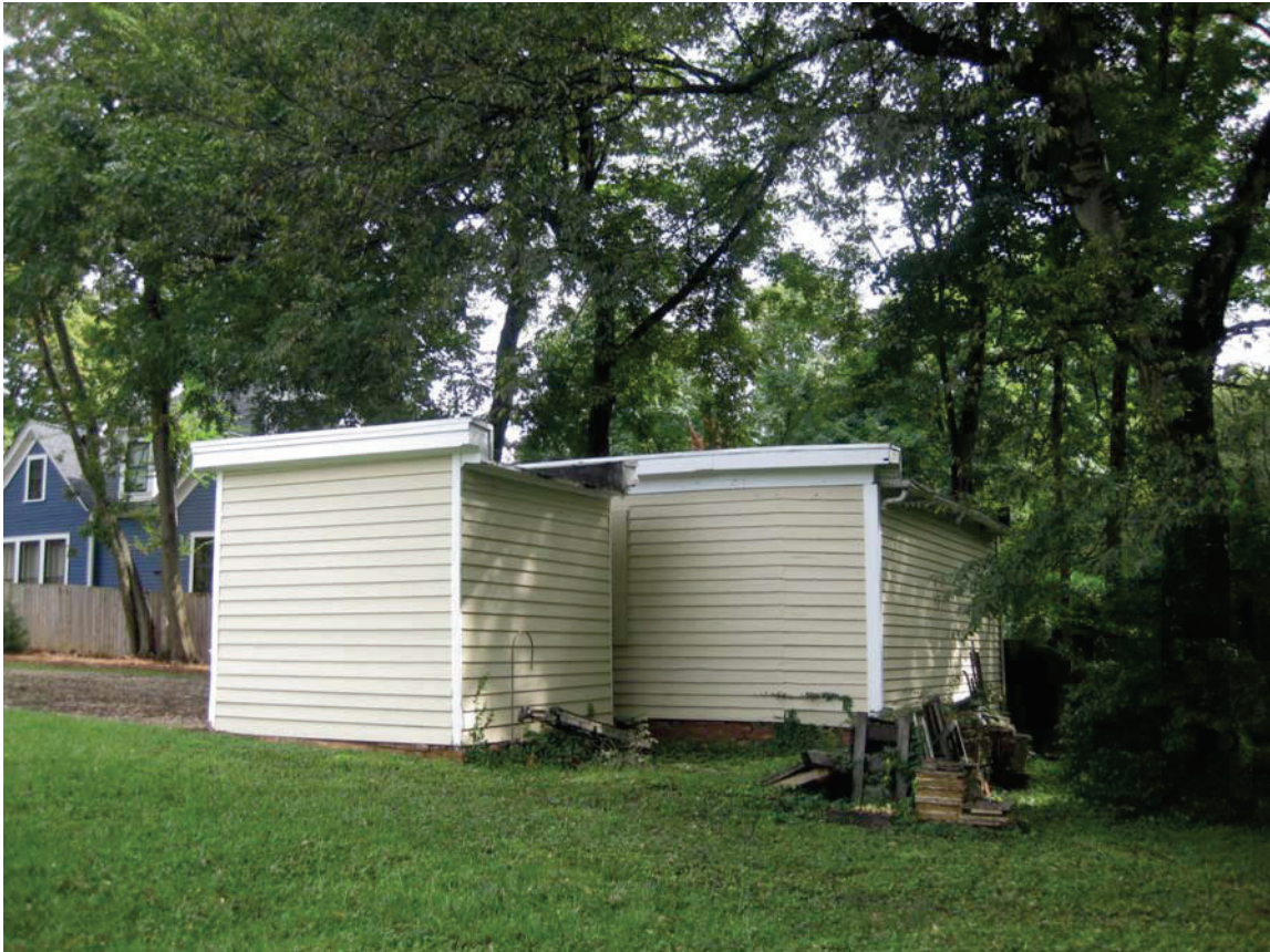
7 Shed and Garage
