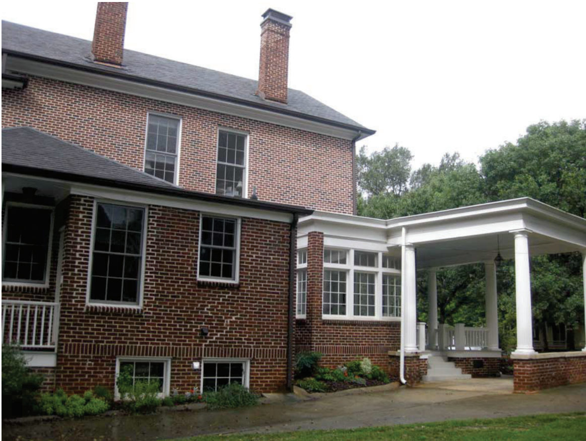
3 Exterior East Elevation
