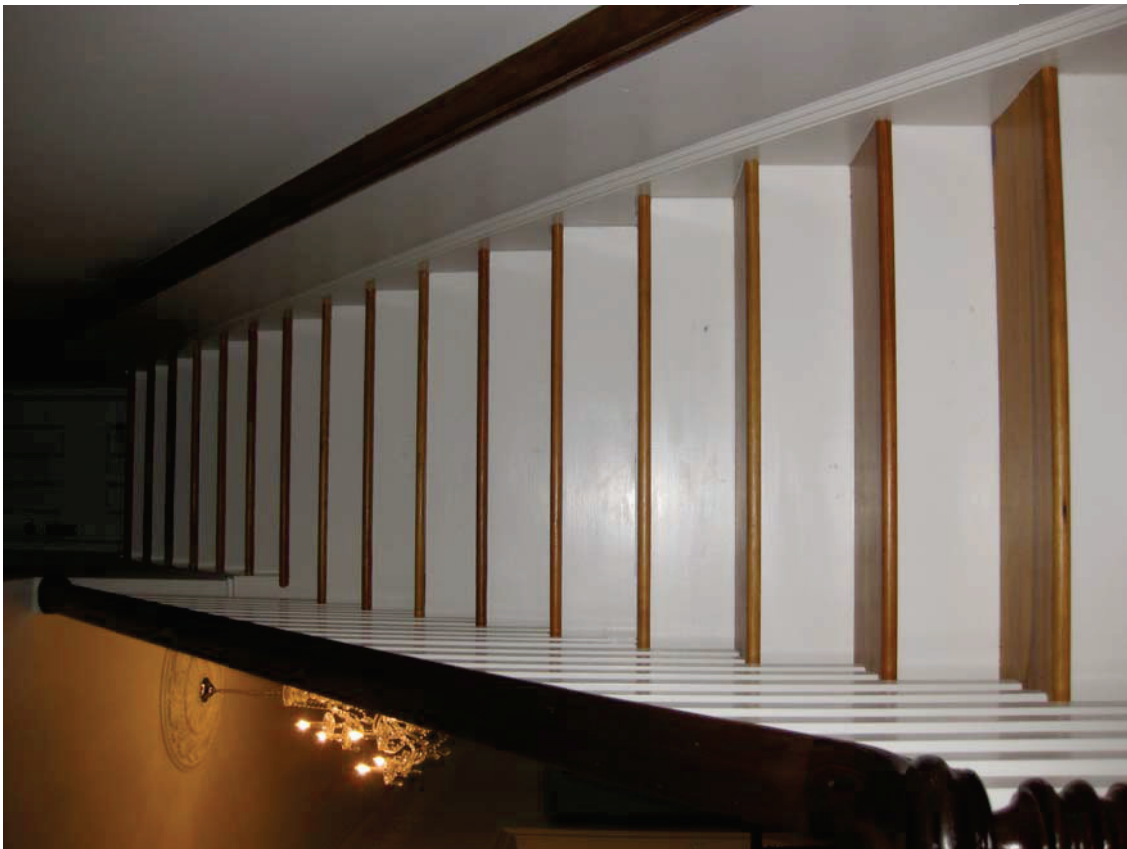
30 Interior Second Floor stairs to attic
