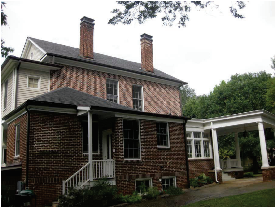
4 Exterior East Elevation
