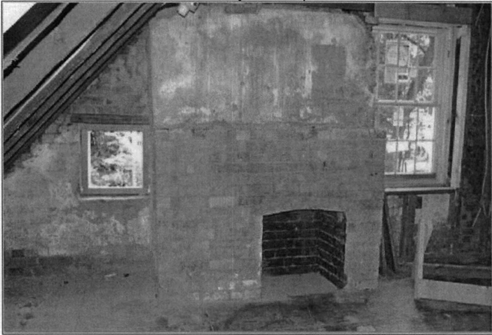
Second story east fireplace
