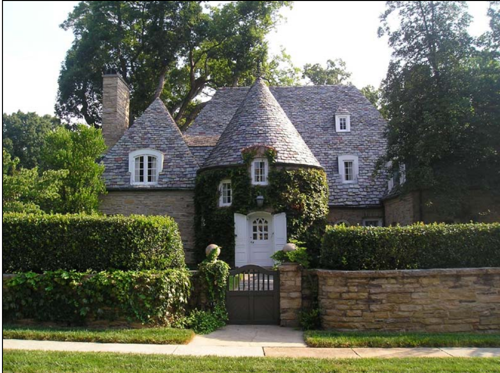
Façade from Harvey Street
