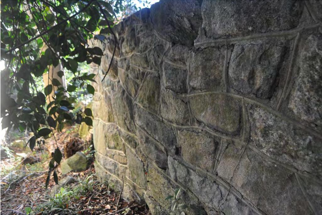
Plate 31: View of the garden showing a four-foot-tall mortared rock wall along the west perimeter.
