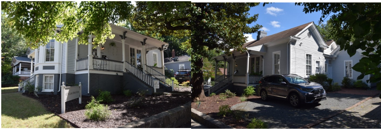
220 N. Boylan Ave. at SE corner with W. Lane St. Photo on left is oblique view of north elevation and façade with camera pointing SE. Photo on right is oblique with façade and S elevation with camera pointing NE.
