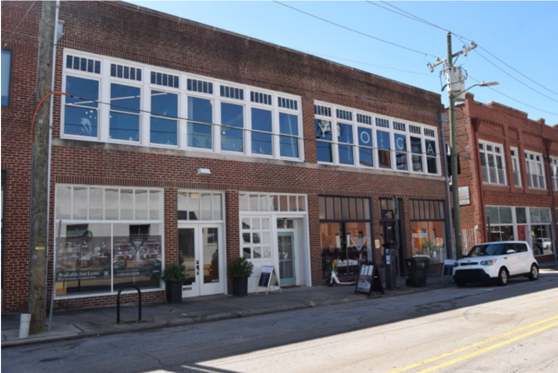
307-309 W. Martin St., White Rabbit Books and Things occupied the storefront on the right; The Front Page newspaper production office was in the back of the space. View to SW.
