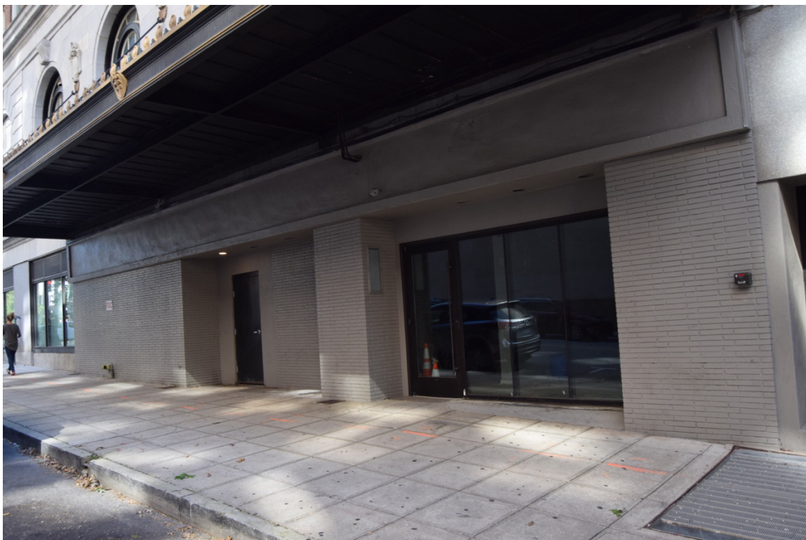
Sir Walter Raleigh Hotel, 400 Fayetteville St., W. Davie St. elevation below canopy, view to NE.
