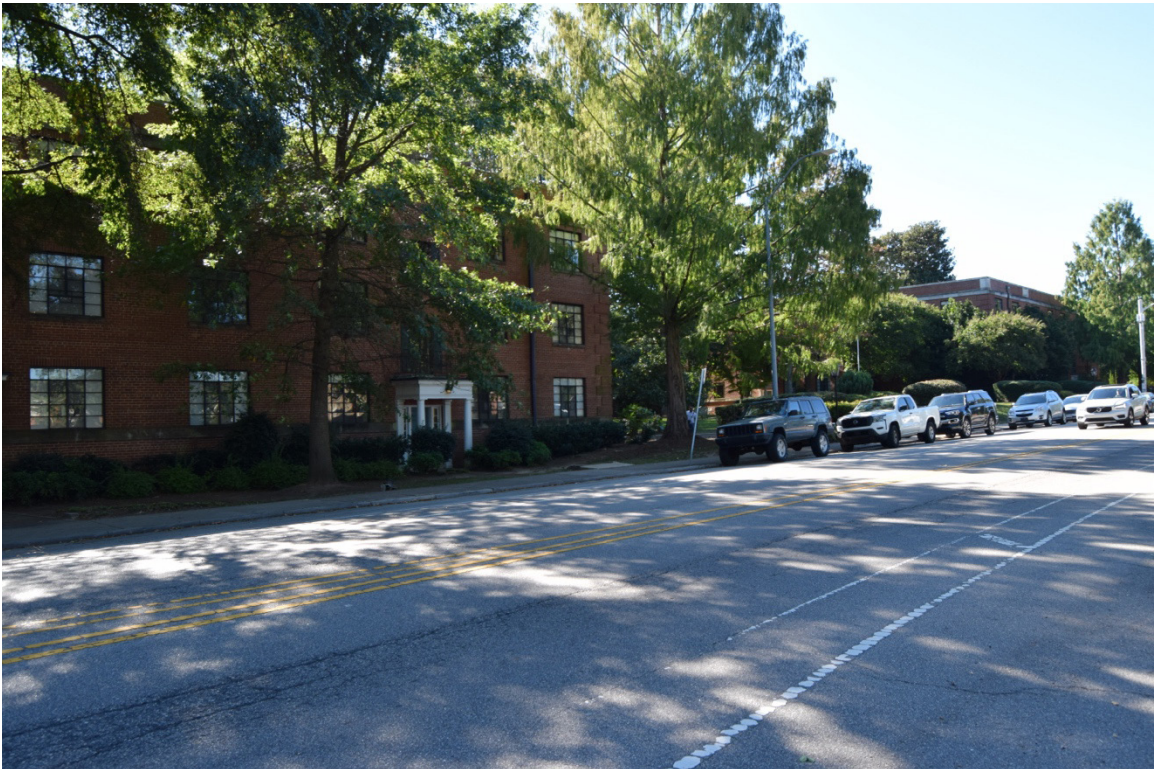
Cameron Court, 905 Hillsborough St., apartment buildings at Hillsborough St., view to SW near NE corner of block.
