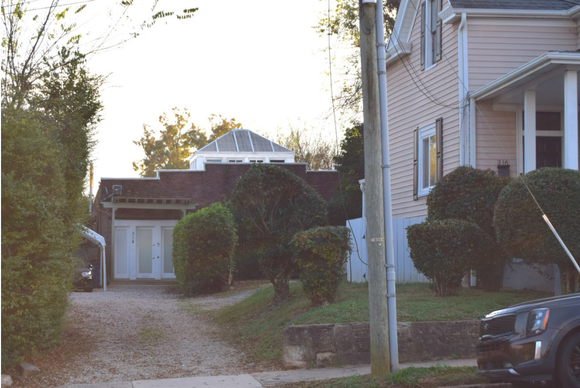
(former) J. C. Raulston House, 318 E. Davie St.
