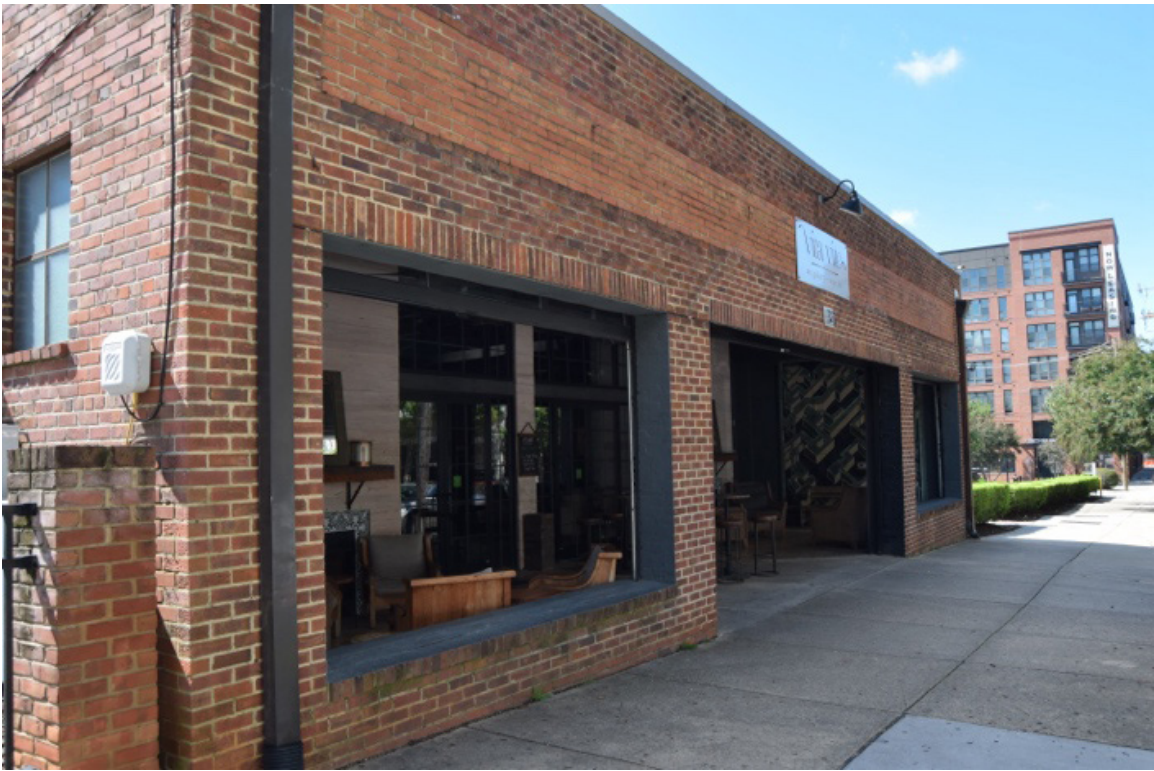
(former) Capital Corral, 313 W. Hargett St., façade, view to SW.
