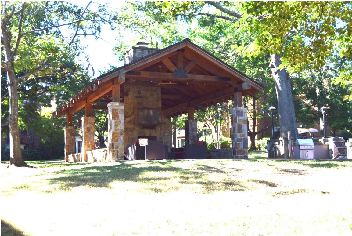
Cameron Court, 905 Hillsborough St., view to NE of pavilion and patio near S. end of quadrangle.
