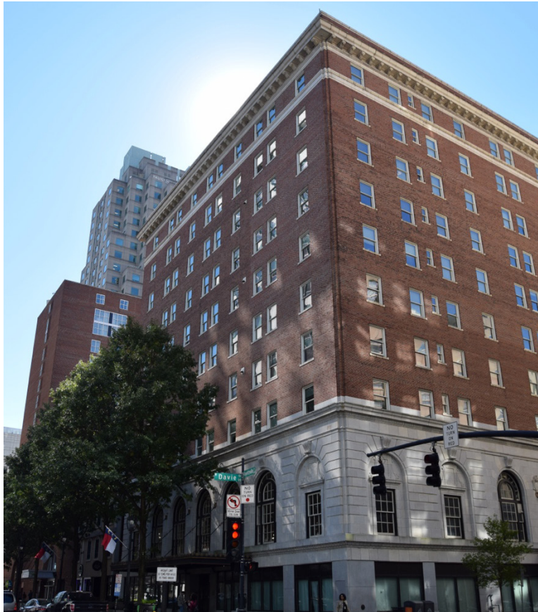
Sir Walter Raleigh Hotel, 400 Fayetteville St., façade and W. Davie St. elevation, view to SW.
