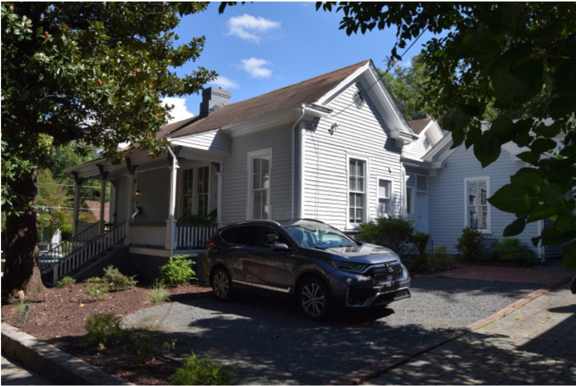
220 N. Boylan Ave., oblique view of façade and S. elevation with camera facing NE.
