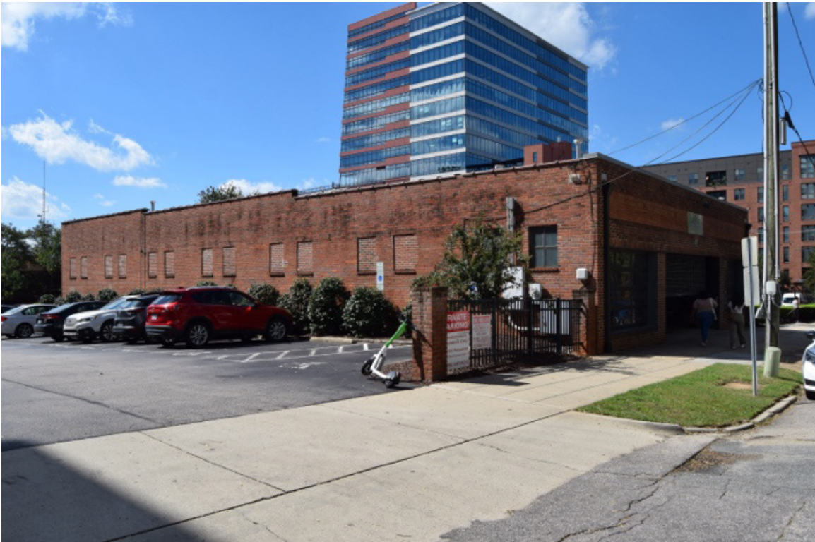
(former) Capital Corral, 313 W. Hargett St. E. elevation and façade, view to SW.
