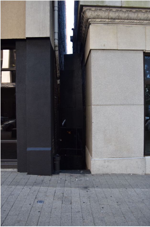
Sir Walter Raleigh Hotel, 400 Fayetteville St., Alley between Sir Walter Raleigh Hotel (r) and neighboring building, view W.
