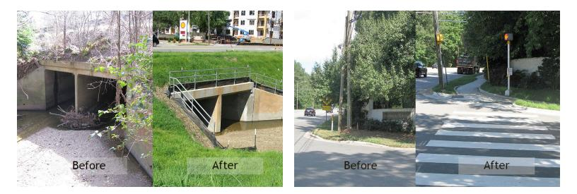
The **Six Forks Road Sidewalk Grant** provides new sidewalk on the north side of the road from Wake Forest Road to Coleridge Road, and a box culvert extension at Big Branch.
