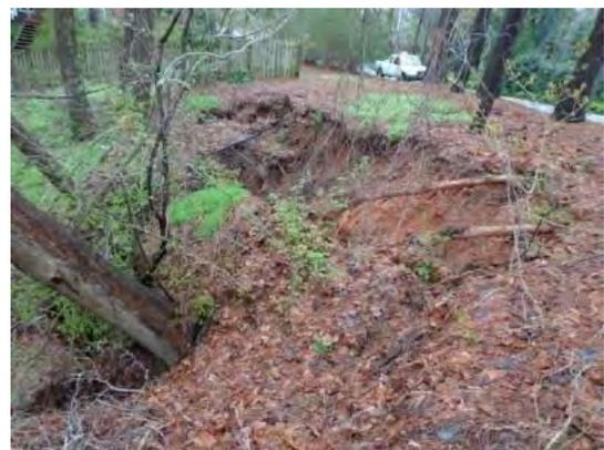
This category includes culvert and stormwater system repairs such as Blenheim Drive (pictured at right), where a large tree situated above the culvert fell causing five sections of 54-inch pipe to become separated. Severe erosion occurred along the fill slope above the culvert that threatened the sidewalk and roadway.
