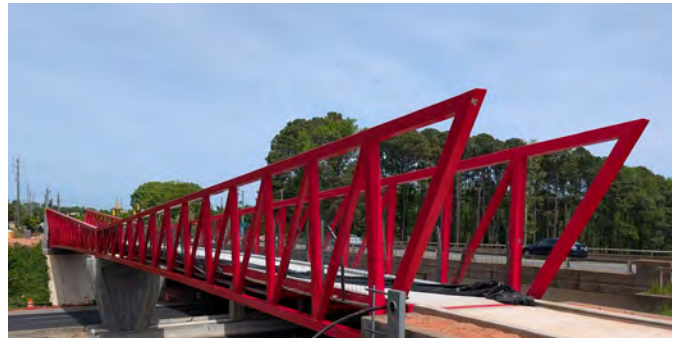
Blue Ridge Road Bike and Pedestrian Bridge
