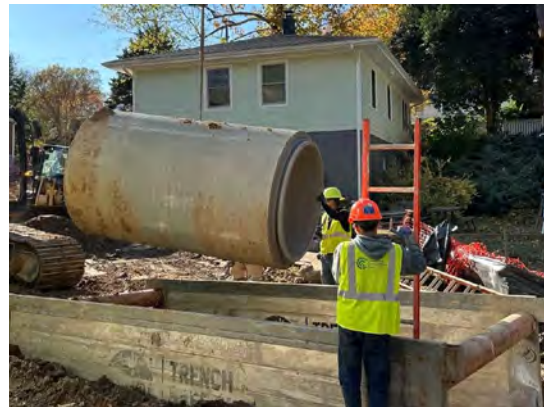
North Boundary Street Emergency Repair
