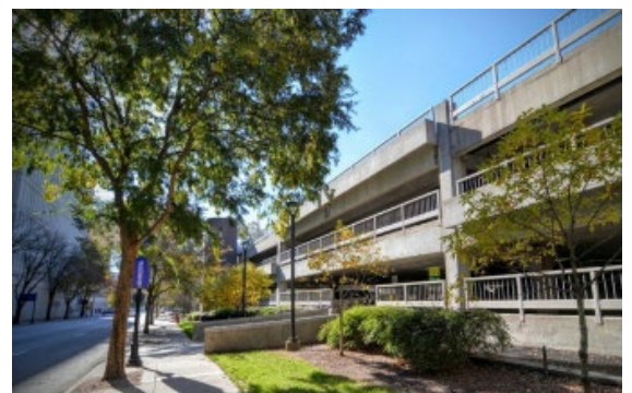
Raleigh Municipal Parking Deck
