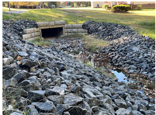
Sierra Drive Capital Improvement Project
