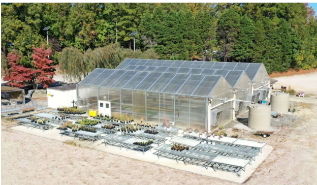
Cisterns at Marsh Creek Park Greenhouse installed through Raleigh Rainwater Rewards
