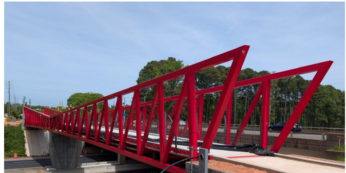
Blue Ridge Road Bike and Pedestrian Bridge
