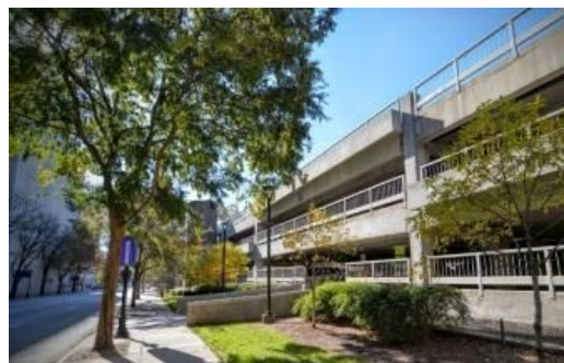
Raleigh Municipal Parking Deck
