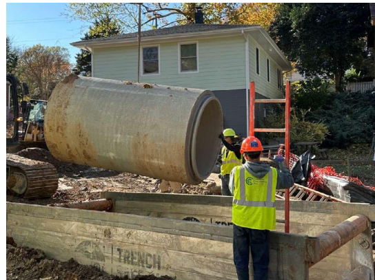
North Boundary Street Emergency Repair
