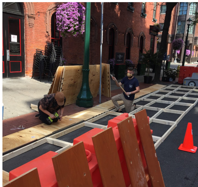
Pressure-treated wood or composite lumber framing. A wood frame for a streetery under construction. Credit: syracuse.com
