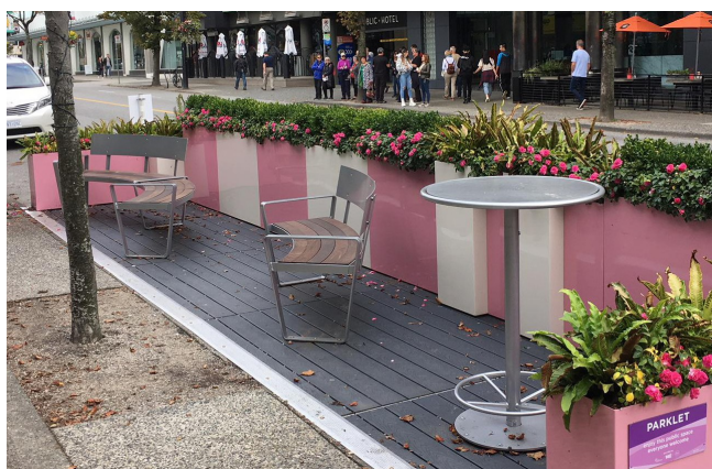
Plastic or composite lumber. An example of decking made from plastic lumber. Credit: montgomeryplanningboard.org
