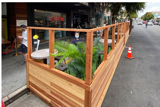
G5.1.4 Mid-range enclosure materials. Top: Planters and railings made of aluminum, Credit: dwell.com. Bottom: A natural wood enclosure surrounds seating, Credit: parkade.com
