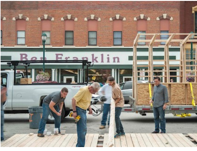
Wood decking is installed over a wooden frame. Substructure joists run parallel to the street. Credit: askstudio.com
