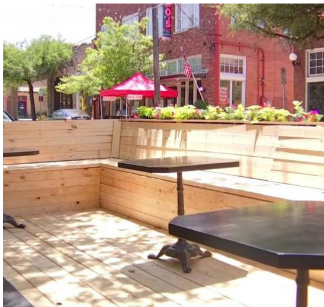
Pressure-treated wood. An example of a streetery deck constructed with wood. Credit: orcity.org
