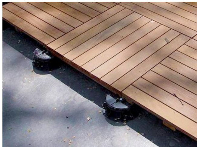
An example of pedestals supporting specialty wooden deck tiles. Credit: decksdirect.com
