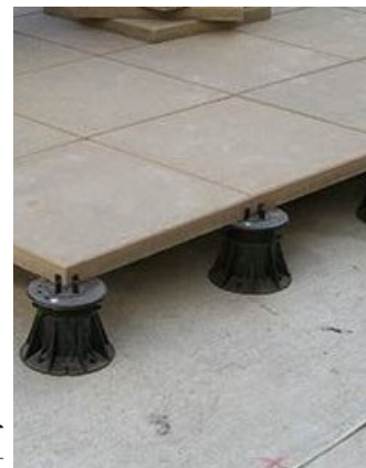
Pedestal support system. Left: A diagram detailing a pedestal support unit. Right: Pedestals supporting concrete pavers. Credit: speedypavingtexas.com
