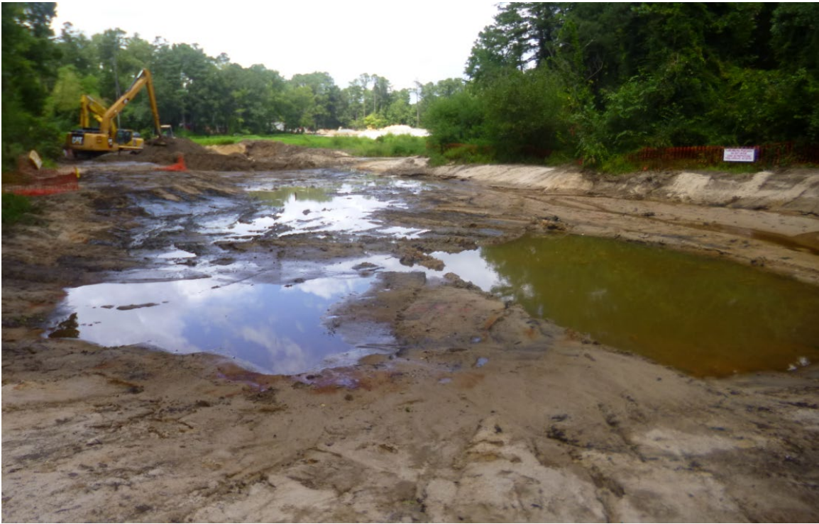
Photo 2. A long-armed excavator removed sediment in the area of the eastern tributary, which was accessed by driving across the lakebed from/to the western tributary access point to Longview Lake Road.
