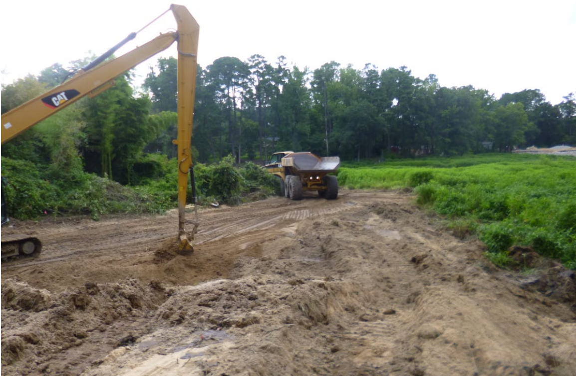
Photo 3. An articulated dump truck backing up to be loaded with sediment by the long-armed excavator. Photo taken near the eastern tributary entrance to the lake.
