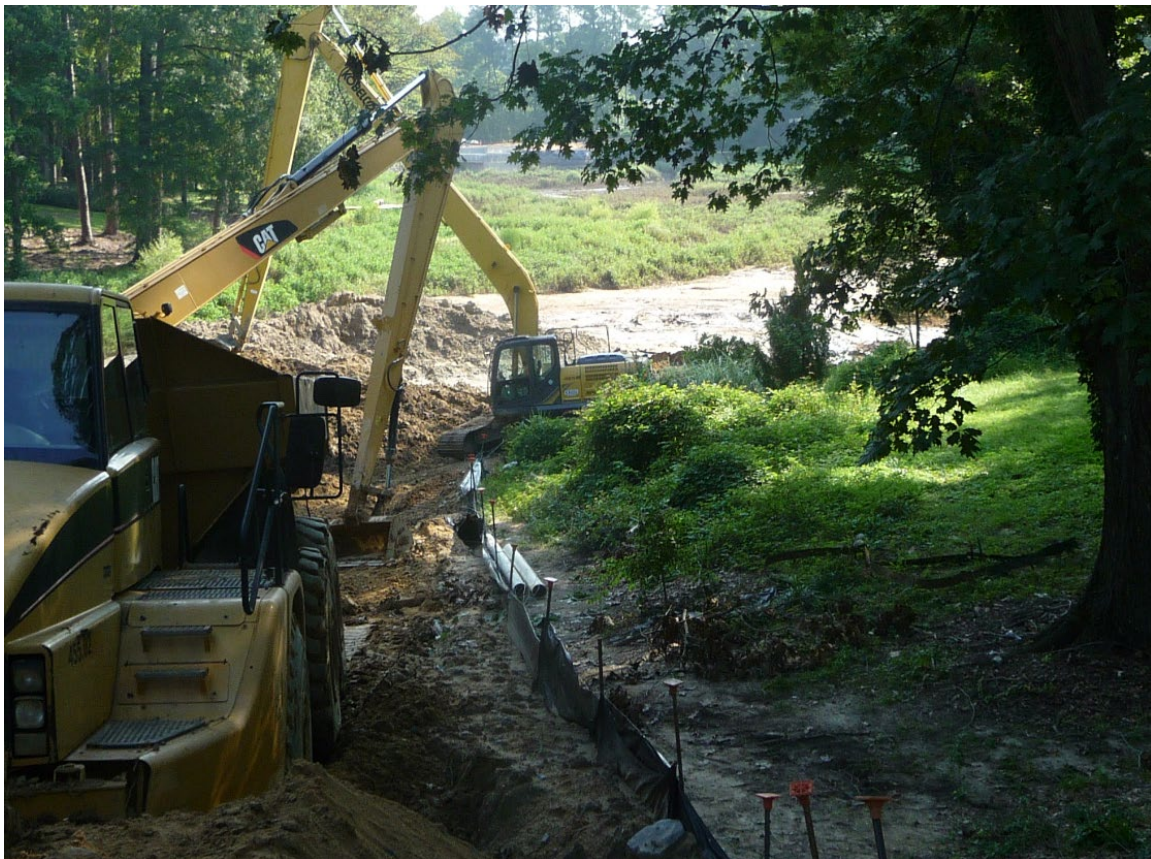
Photo 1. Long-armed excavators remove sediment and load an articulated dump truck for subsequent hauling of the sediment off site. Photo taken near the access point off Longview Lake Road near the western tributary.
