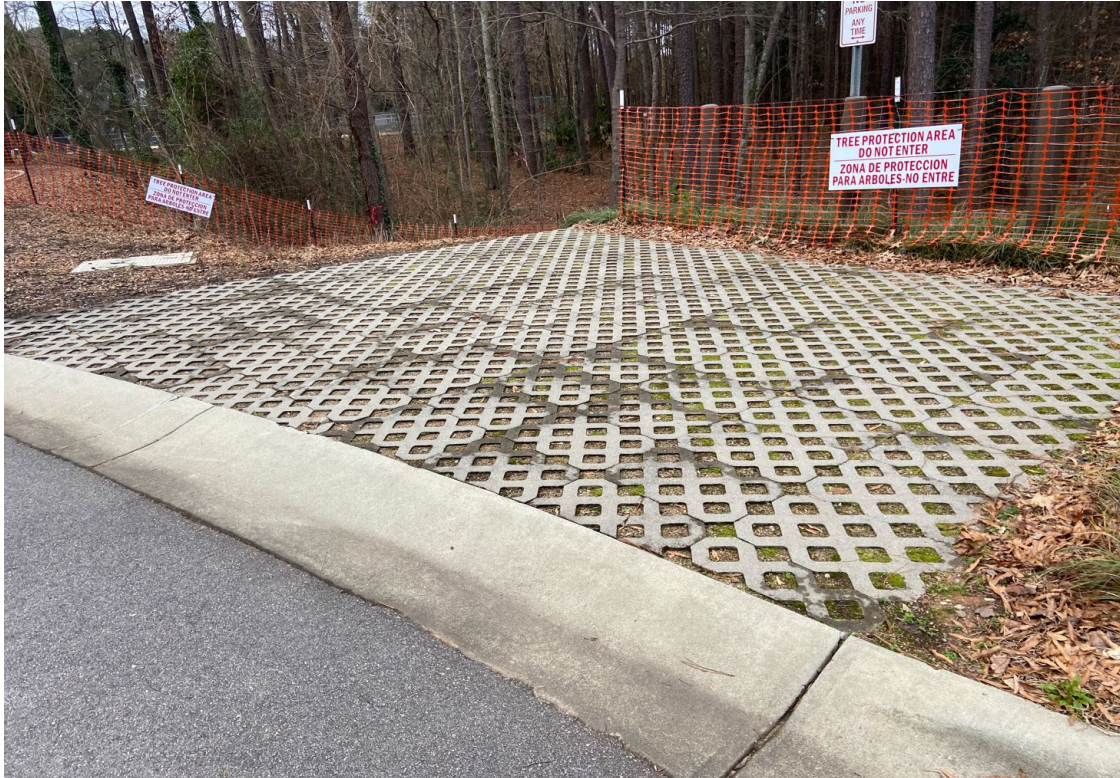
Turnaround pad at Lake Johnson Park Community Center
