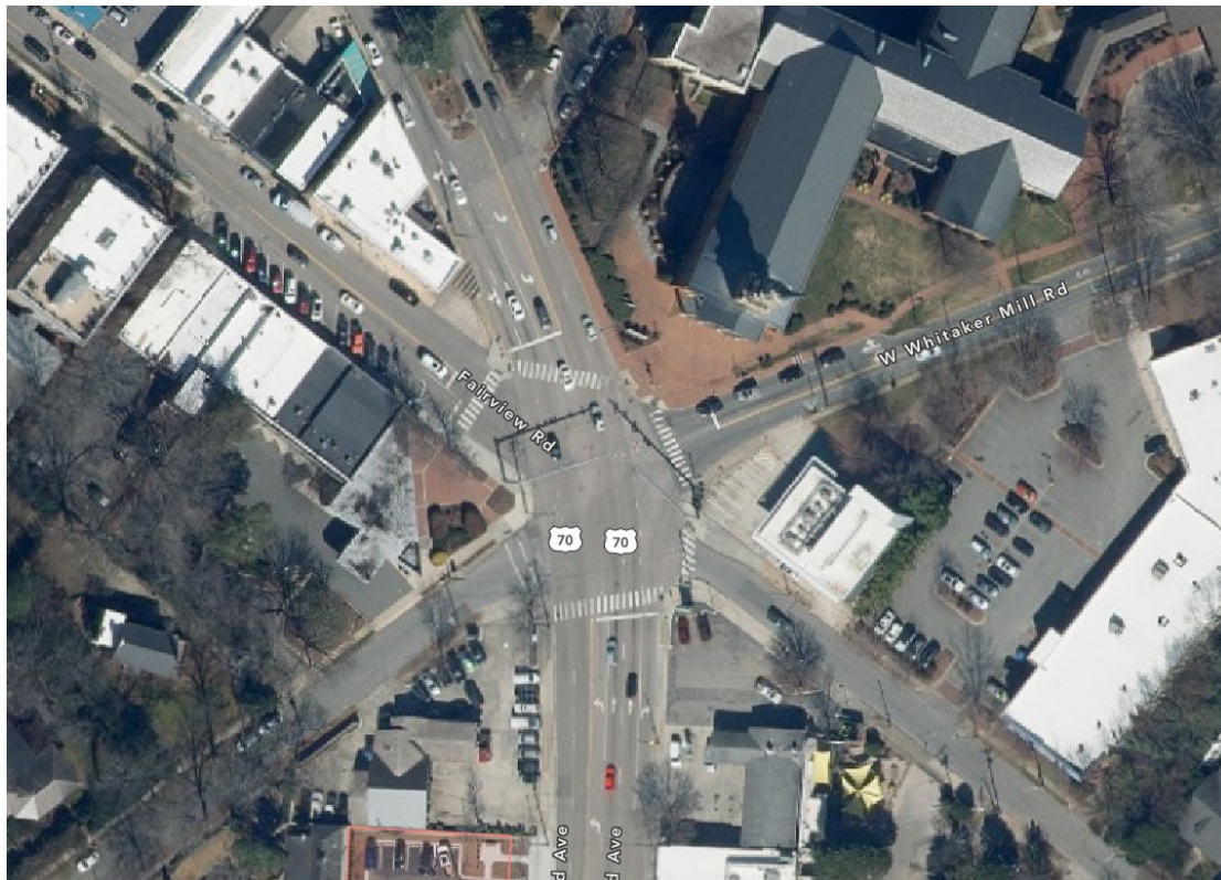
Overhead View of Five Points Intersection
