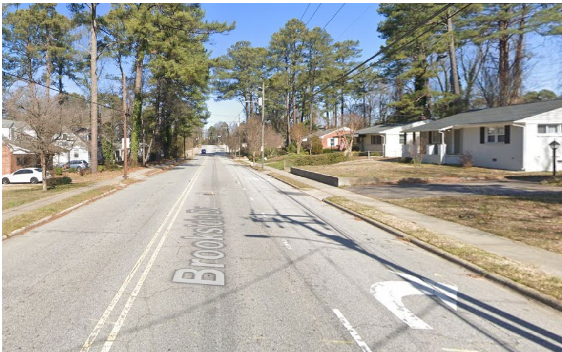
Existing Brookside Drive looking north toward Frank Street/Conn Elementary
