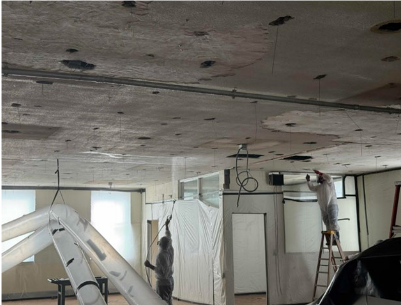
1st Floor Main Building Abatement Ceiling tiles and Grid removal
