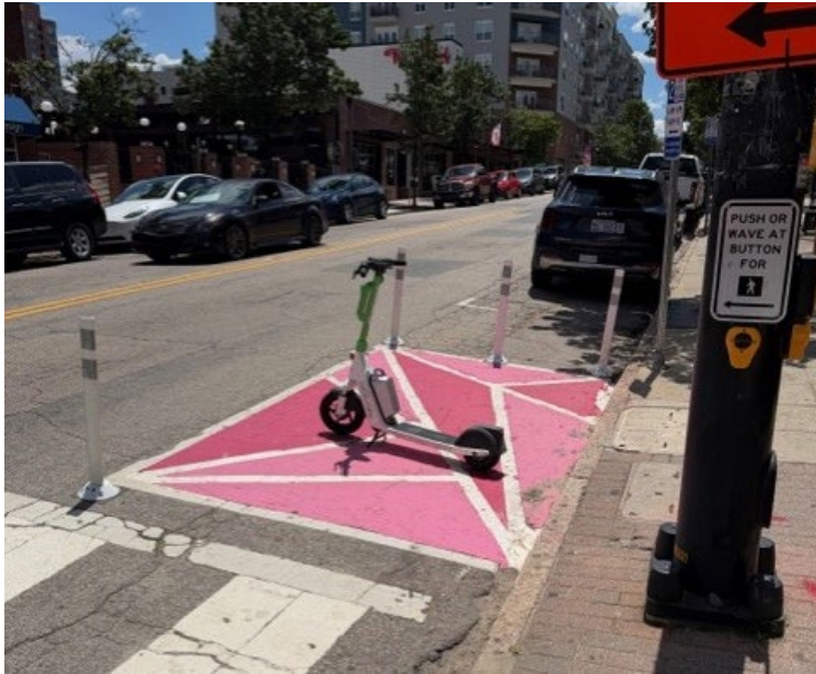
Stage 3: Install Vertical Delineators
