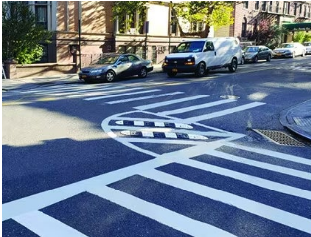
Example of turn calming wedge installation (New York City)
