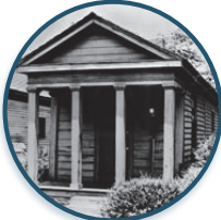
Old Office Building
