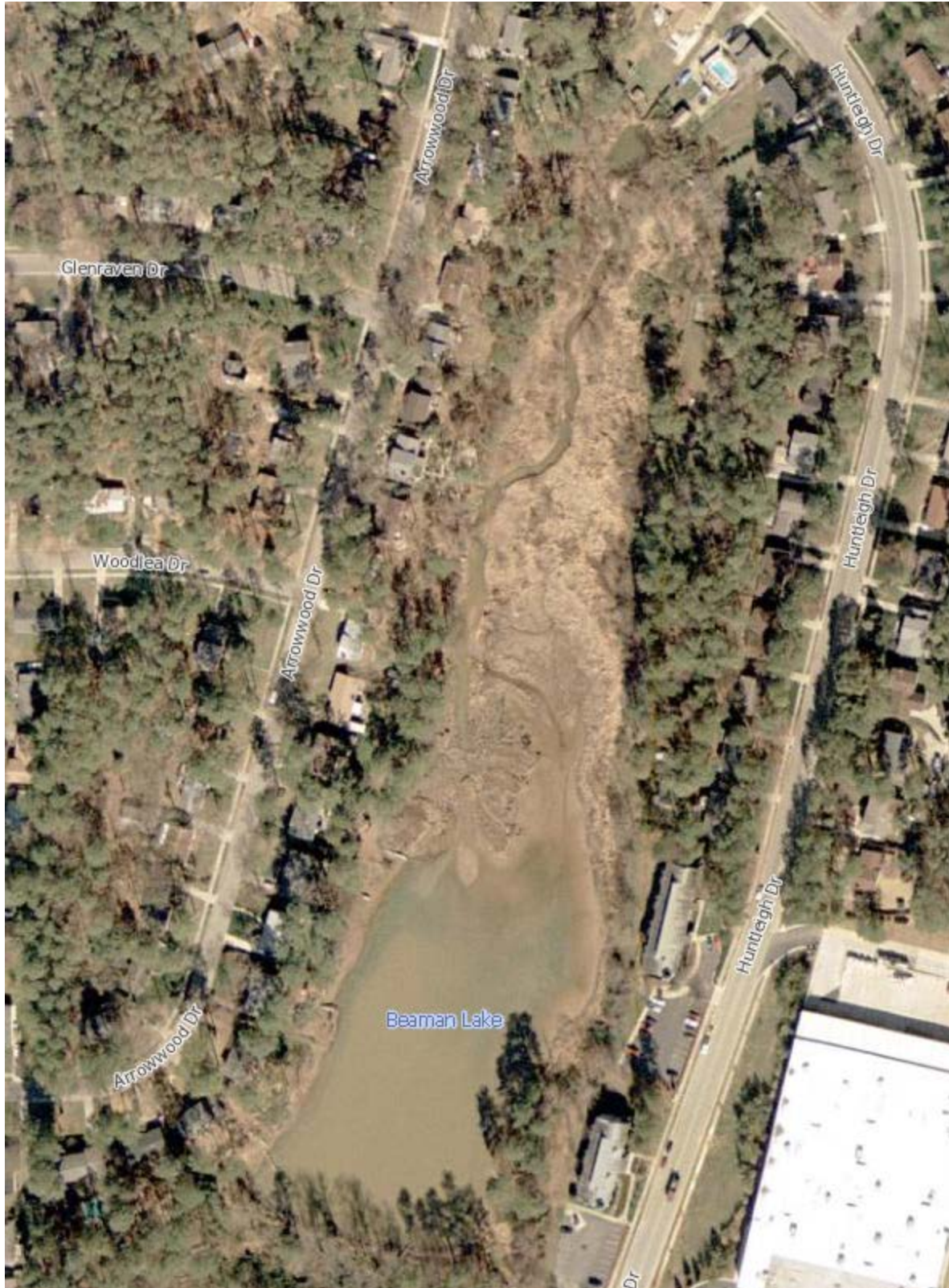
Figure 2. Beaman Lake 1999, after dam failure occurred in the late 1980s.
