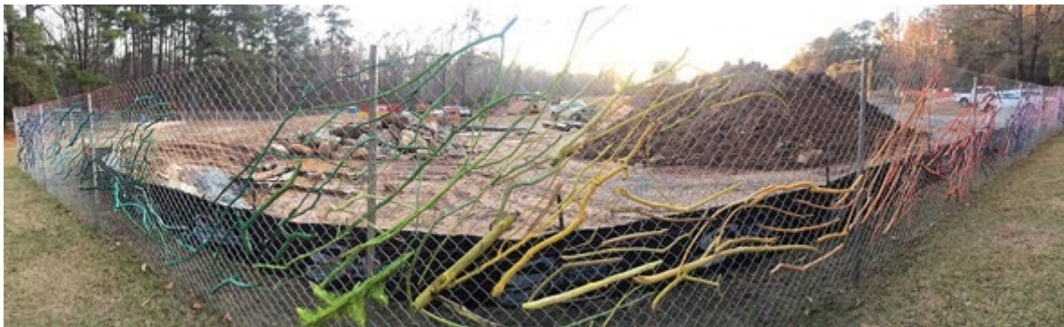
Panorama of Keith Norval and Anna Podris' construction fence installation at Durant Nature Preserve
