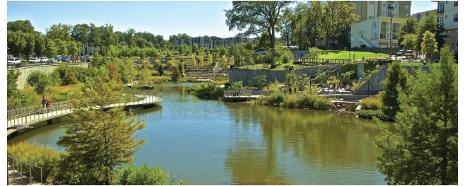
▲ Historic Fourth Ward Park in Atlanta, GA. The park's 2-acre lake also acts as a stormwater retention pond. This design feature solved flooding issues that plagued the Old Fourth Ward. beltline.org
