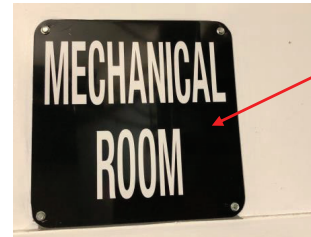
SIGNAGE IS LIMITED IN THE BUILDING. SIGNAGE MISSING BRAILLE.
