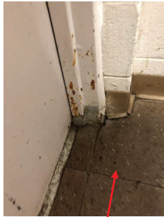
DOOR FRAMES RUSTING AND DAMAGED
