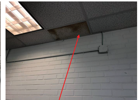
SUSPENDED CEILING DAMAGED
