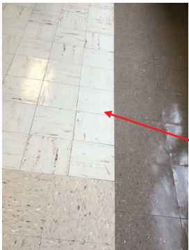
ASBESTOS FLOOR TILES
