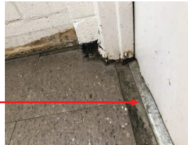
DOOR FRAMES DAMAGED
