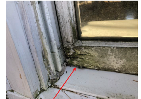
WINDOW FRAMES AND SASHES ARE WEATHER ROTTING
