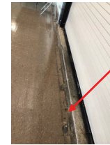
VCT FLOORING DAMAGED
