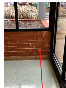
IRREGULAR CRACKING
