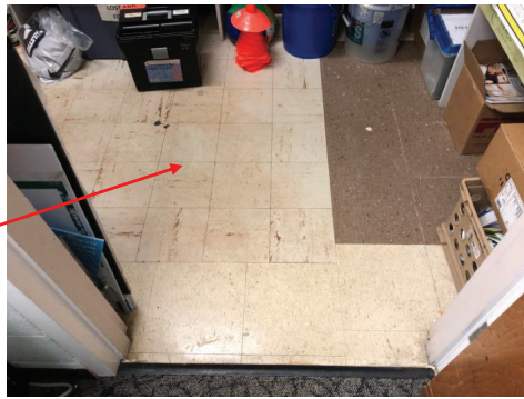
ASBESTOS FLOOR TILES
