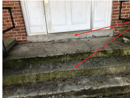
CRACKING IN THE CONCRETE STEPS AND STOOP.
