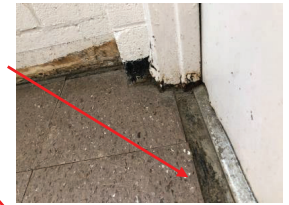
VCT FLOORING DAMAGED
