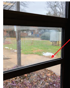
EXISTING GLAZING WITH BROKEN THERMAL SEAL
