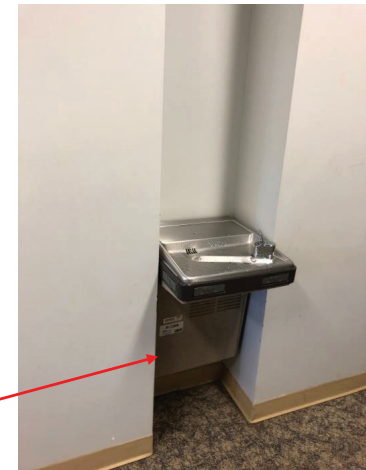
ELECTRIC WATER COOLER DOES NOT PROVIDE ADEQUATE TOE CLEARANCE.
