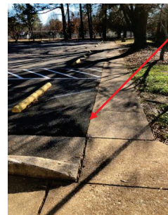
ACCESSIBLE PATH BETWEEN BUILDINGS ON SITE PROVIDE AN IRREGULAR FINISH BETWEEN PARKING AND SIDEWALK
