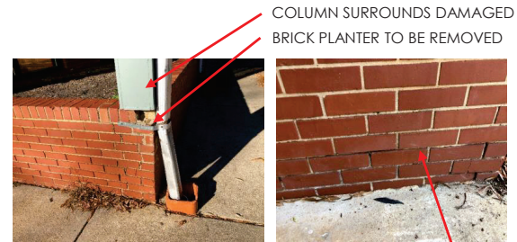
BRICK NEEDS TO BE REPOINTED AND SEALER APPLIED (TYP)
