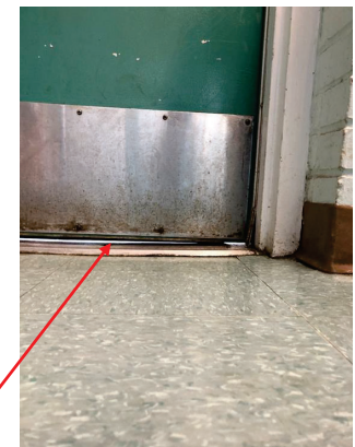
EXTERIOR DOORS LACKING WEATHER- STRIPPING
