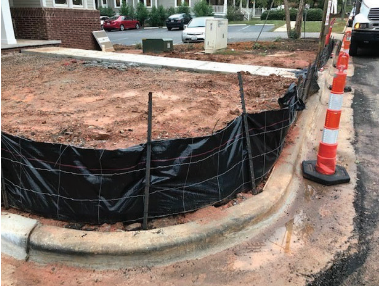
Photograph 1: Silt fence re-installation
