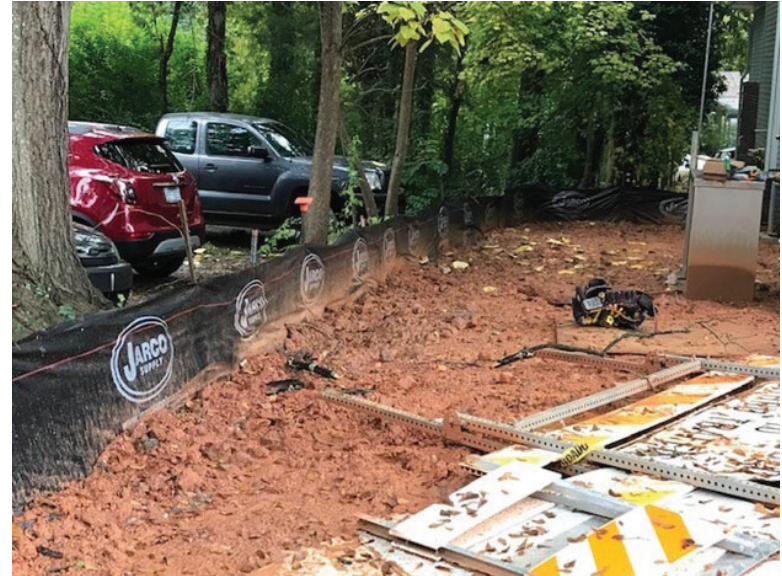
Photograph 2: Side of lot silt fence repairs
