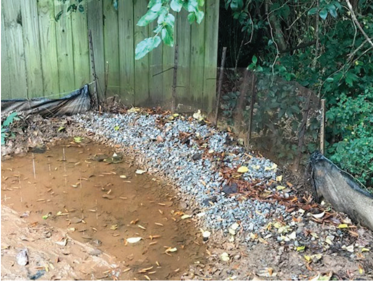
Photograph 3: Silt fence outlet repair
